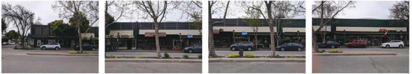
Existing Building East Elevation
