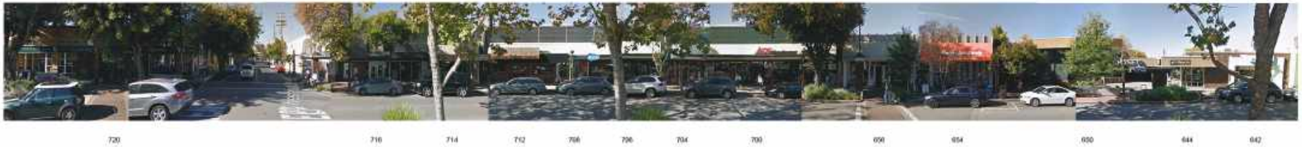
3. Santa Cruz Ave Existing Streetscape
