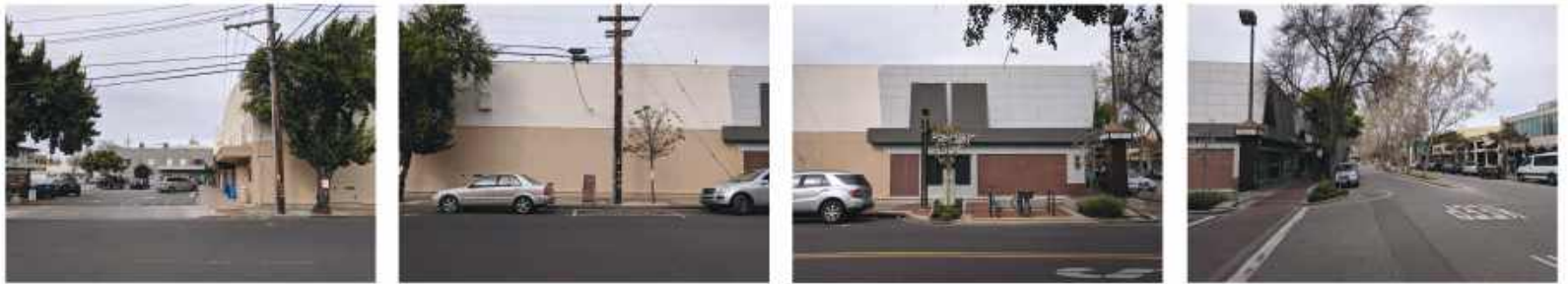
Existing Building South Elevation
