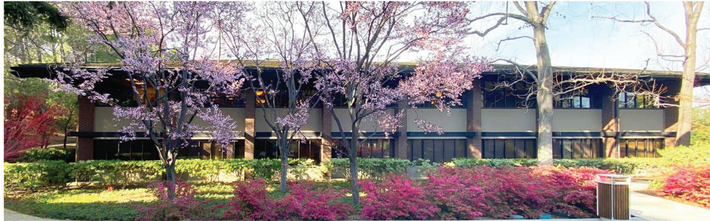
2. (E) BUILDING PHOTO - LEFT - SOUTH
