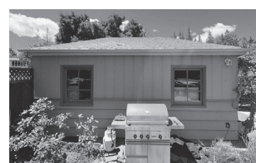
EXISTING GARAGE LEFT SIDE
