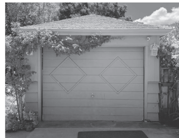
EXISTING GARAGE FRONT
