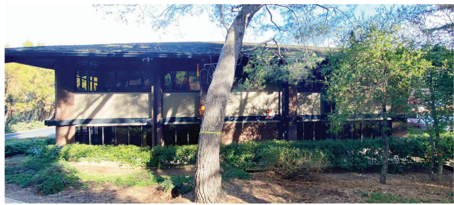
2. (E) BUILDING PHOTO - REAR - WEST
