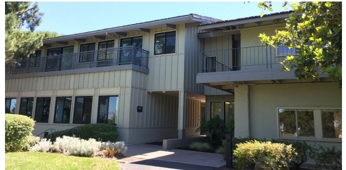
Existing entrance at 2450 (area of work)
