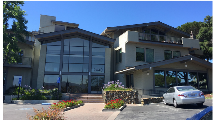
Existing entrance at 2440
