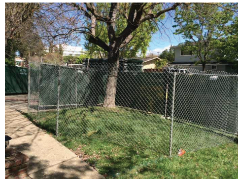
Figure 5: Example of Tree Protection Fencing
