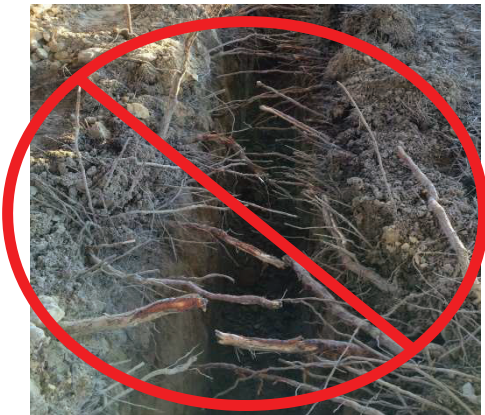
Figure 8: How not to trench
