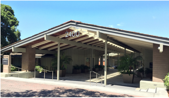
Existing entrance at 2400
