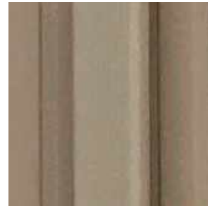
Carport Exposed Metal
