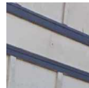
Trim Band at Fitness Building
