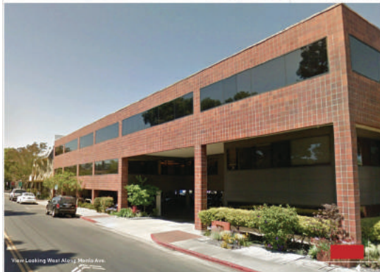
View Looking West Along Menlo Ave.
