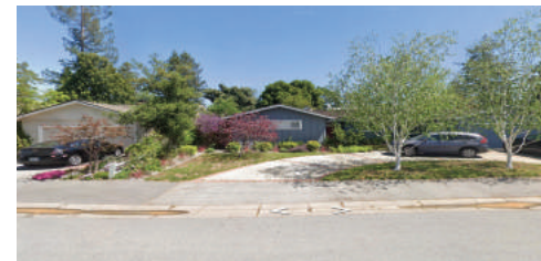
4 EXTERIOR PHOTO OF (E) HOUSE @ 1340 DELFINO WAY FRONT VIEW
