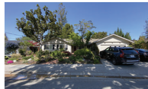
3 EXTERIOR PHOTO OF (E) HOUSE @ 1350 DELFINO WAY FRONT VIEW
