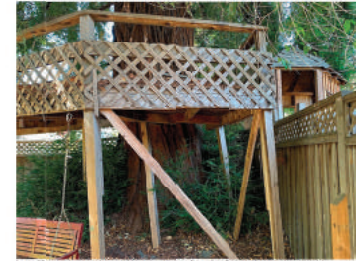
Image #2: Tree T6, coast redwood. Grows near the main house line. Has tree wraps around trunk.
