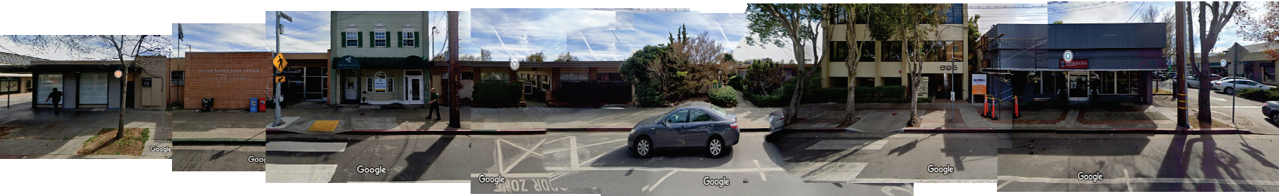
1 PANORAMA - BUILDING SIDE
