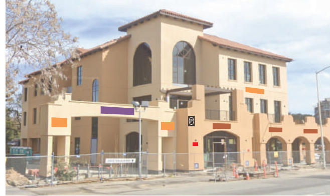
As-built building condition (07-2023)
