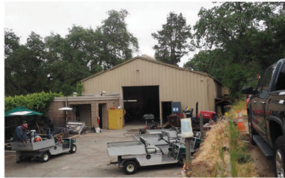
MAINTENANCE BUILDING, NORTH
