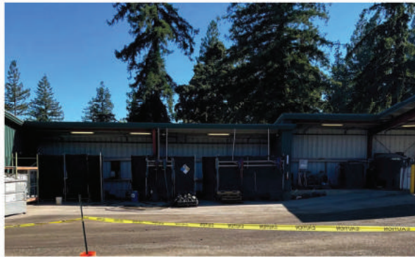
WASH & FUEL STATION, SOUTH
