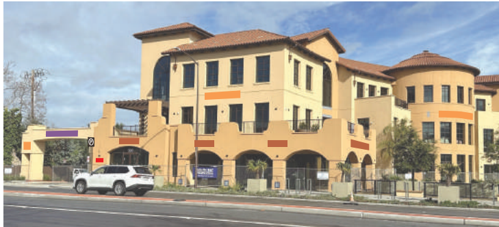
As-built building condition (01-24-2023)
