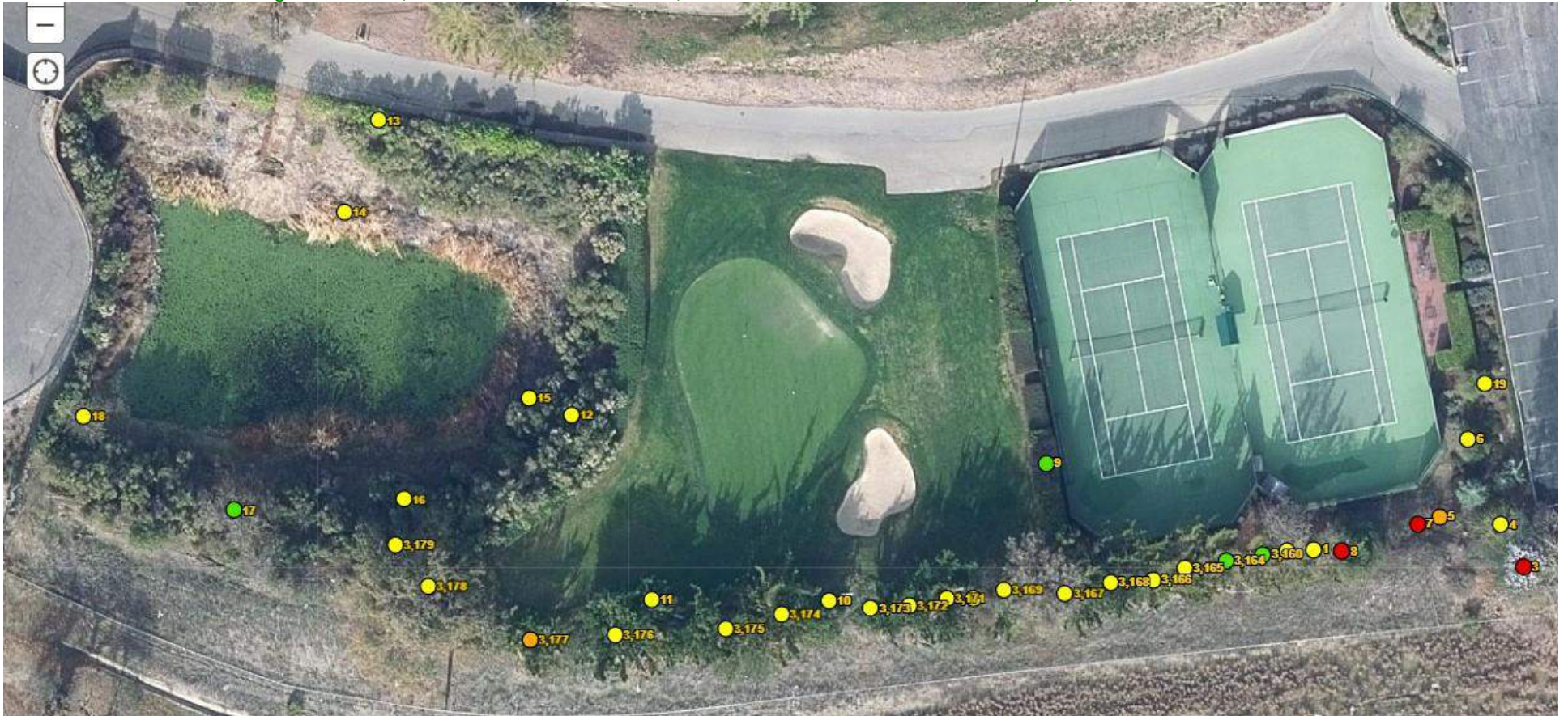
ENLARGED AERIAL W TREE #S IN APPROXIMATE LOCATIONS, #3 IS THE CELL TOWER
