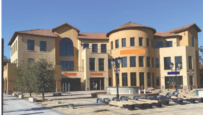
As-built building condition (04-26-2023)
