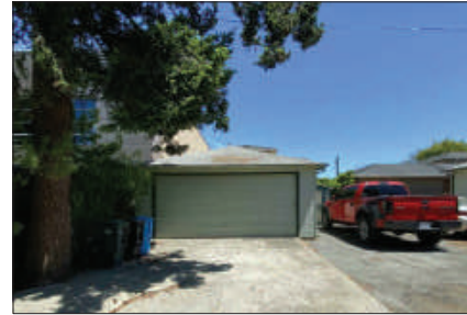
GARAGE 2: REAR SIDE OF PROPERTY (NORTH EAST CORNER) ACCESS FROM HOOVER ST. ON LEFT SIDE OF PROPERTY
