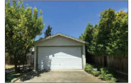
GARAGE 1: RIGHT SIDE AND MIDDLE PART OF PROPERTY, ACCESS FROM HOOVER ST. ON RIGHT SIDE OF PROPERTY
