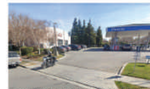
7 - CONVENIENCE STORE AND CANOPY LOOKING SOUTH
