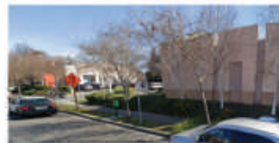
11 - CONVENIENCE STORE AND CARWASH LOOKING SOUTH
