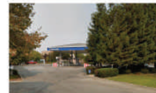
1 - CANOPY LOOKING NORTH
