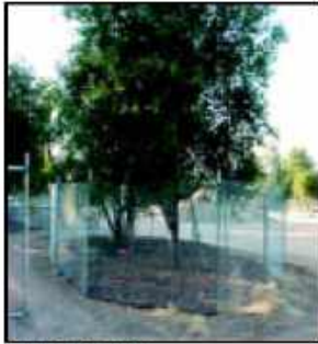
IMAGE 2.15-1 Tree Protection Fence at the Dripline
