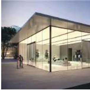
1 BUTT GLAZED CURTAIN WALL REFERENCE IMAGE: CRL
