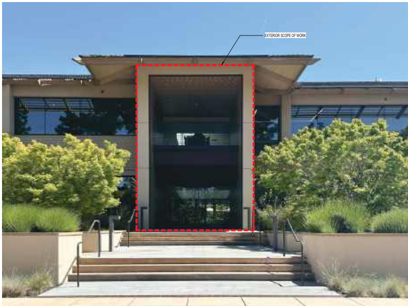
EXISTING EXTERIOR CONDITION: ENTRANCE
