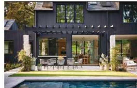
DARK SIDING/STAINED TELLIS/COBBLESTONES/STONE COLUMNS
