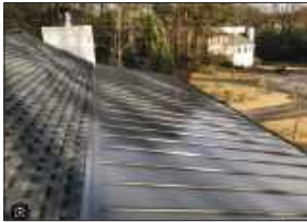
(0) Porch Roof - Standing Seam Metal Roof - Grey
