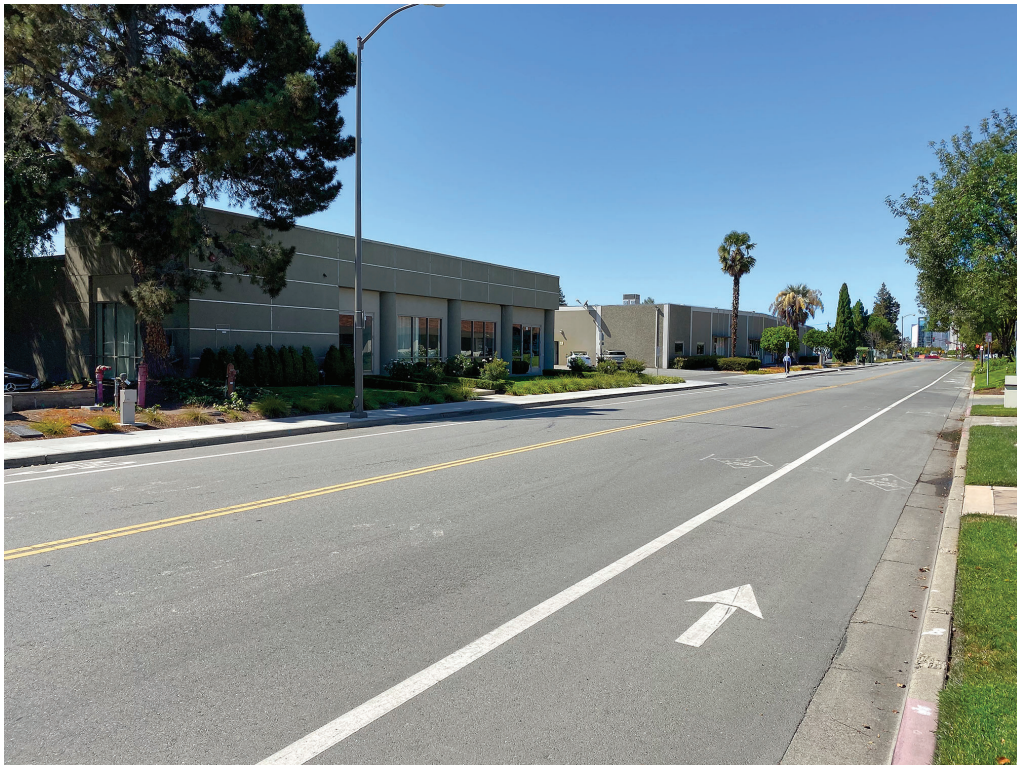
Photo 2: Existing buildings at 180 and 188 Constitution Drive, as seen from Constitution Drive
