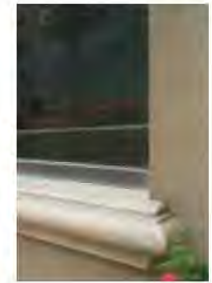
CAST STONE WINDOW SILL
