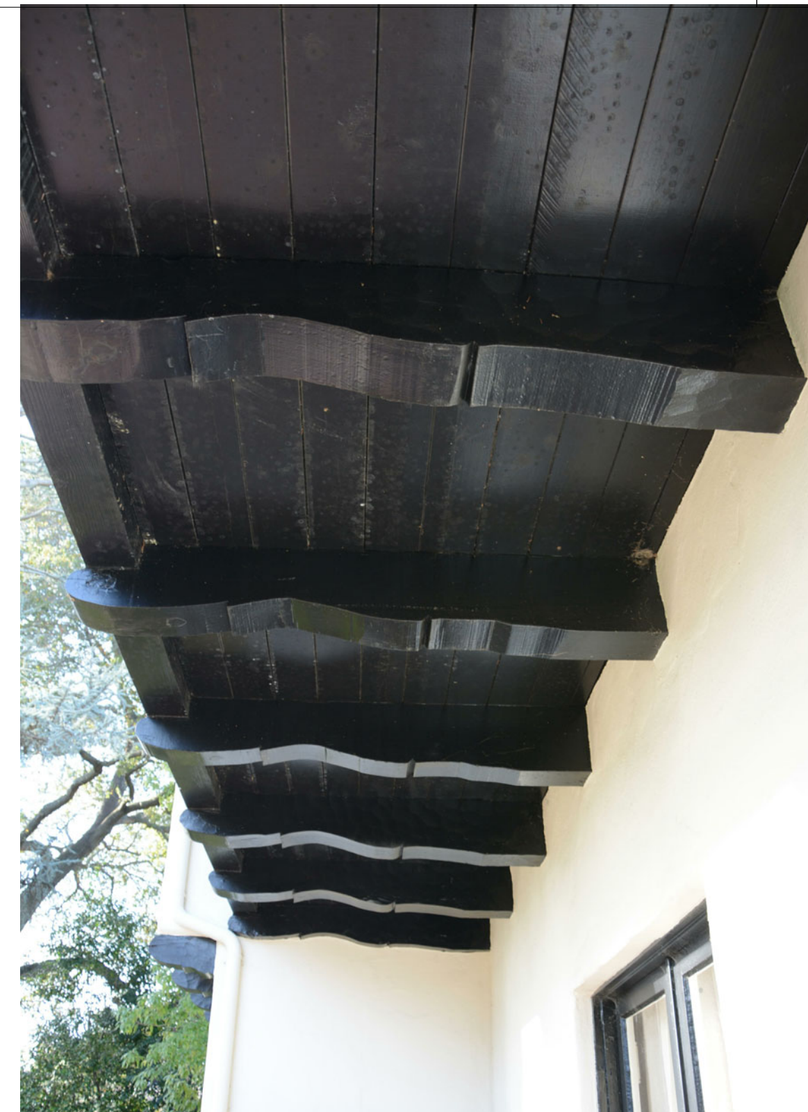
CORBELS UNDER BALCONY 8.
