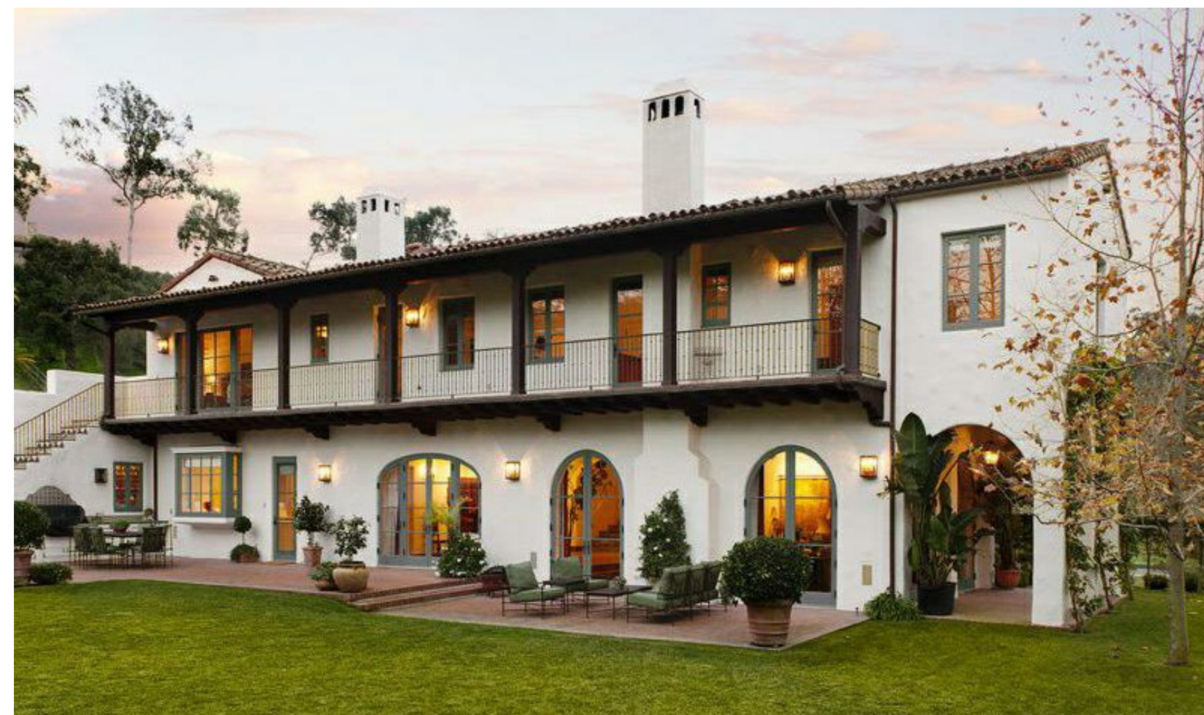
SECOND FLOOR BALCONY WITH POSTS AND THIN RAILINGS, ARCHED WINDOWS/ DOORS, CHIMNEYS 10.
