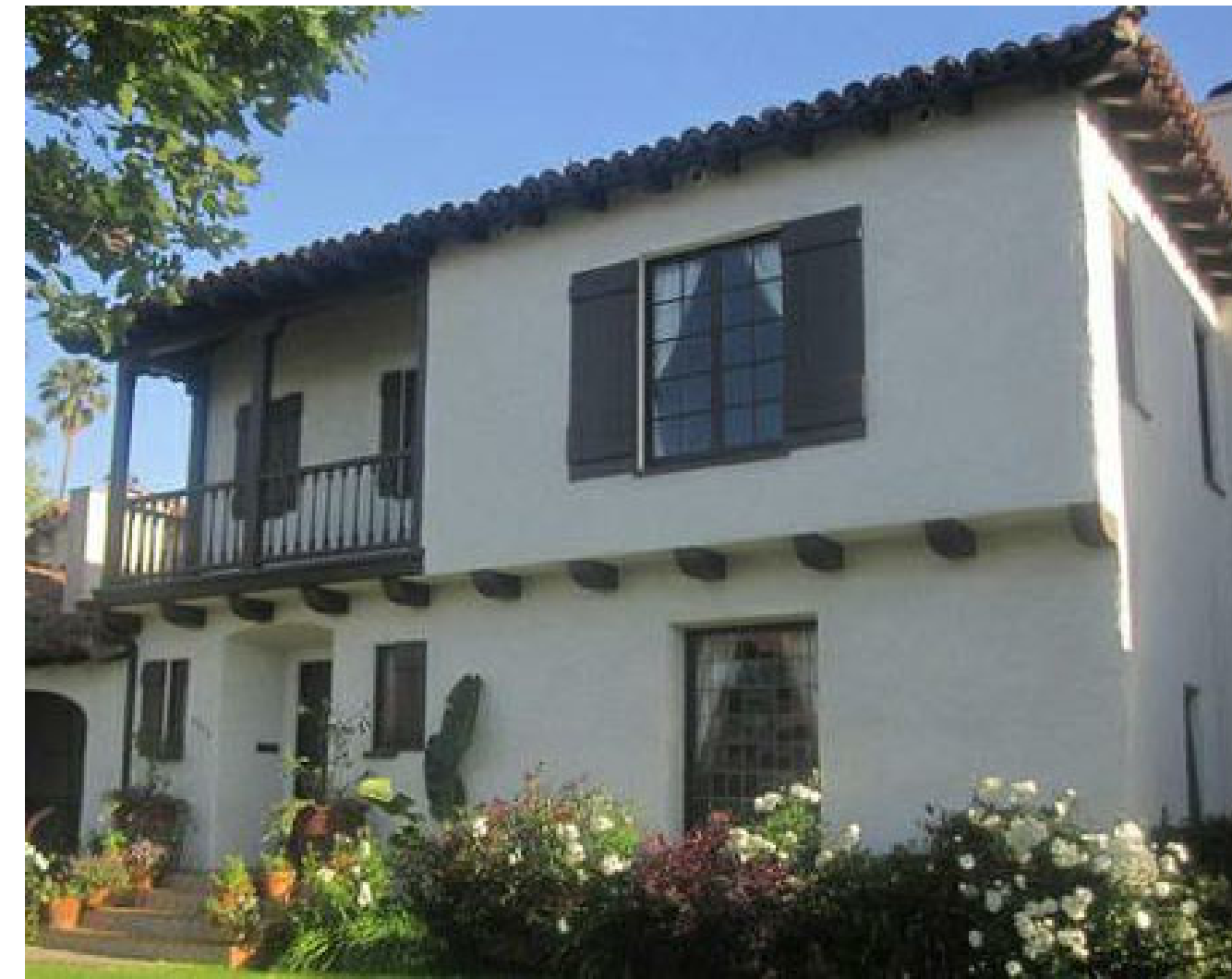
SECOND FLOOR OVERHANG WITH CORBELS 5.
