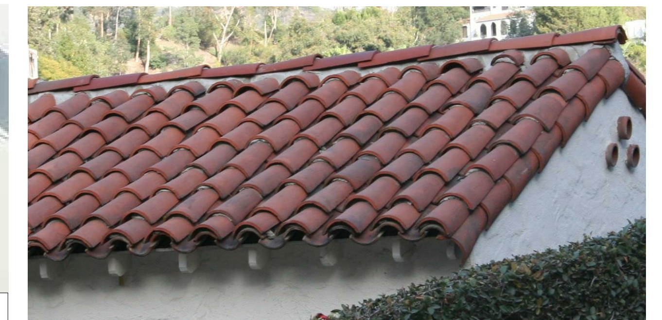
GABLE TILE ROOF WITH VENTS 2.
