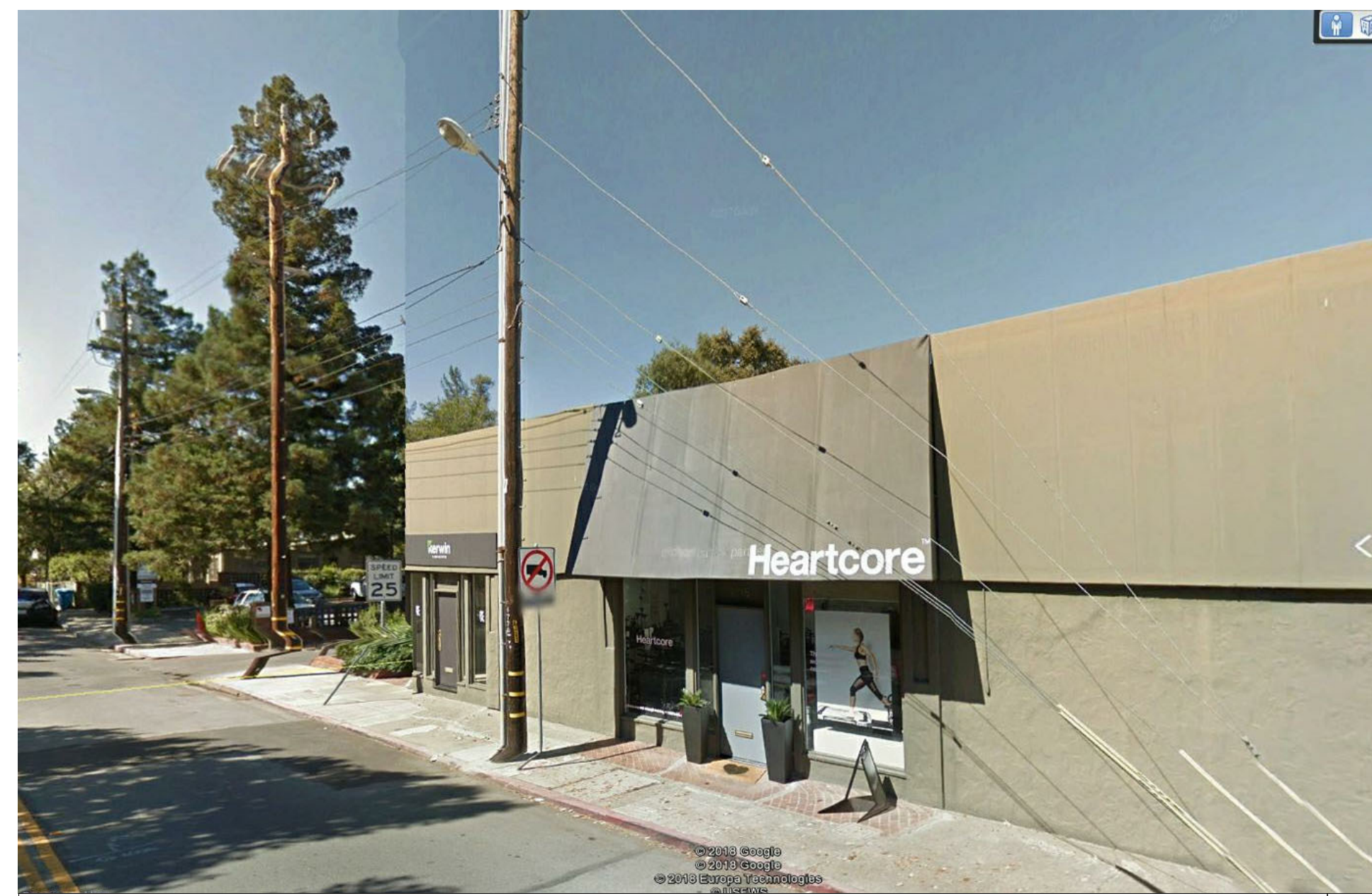
PG&E POLE MOUNTED TRANSFORMER AND AT&T CABLE POLES & GUY WIRES ON CAMBRIDGE AT 201 EL CAMINO 6.
