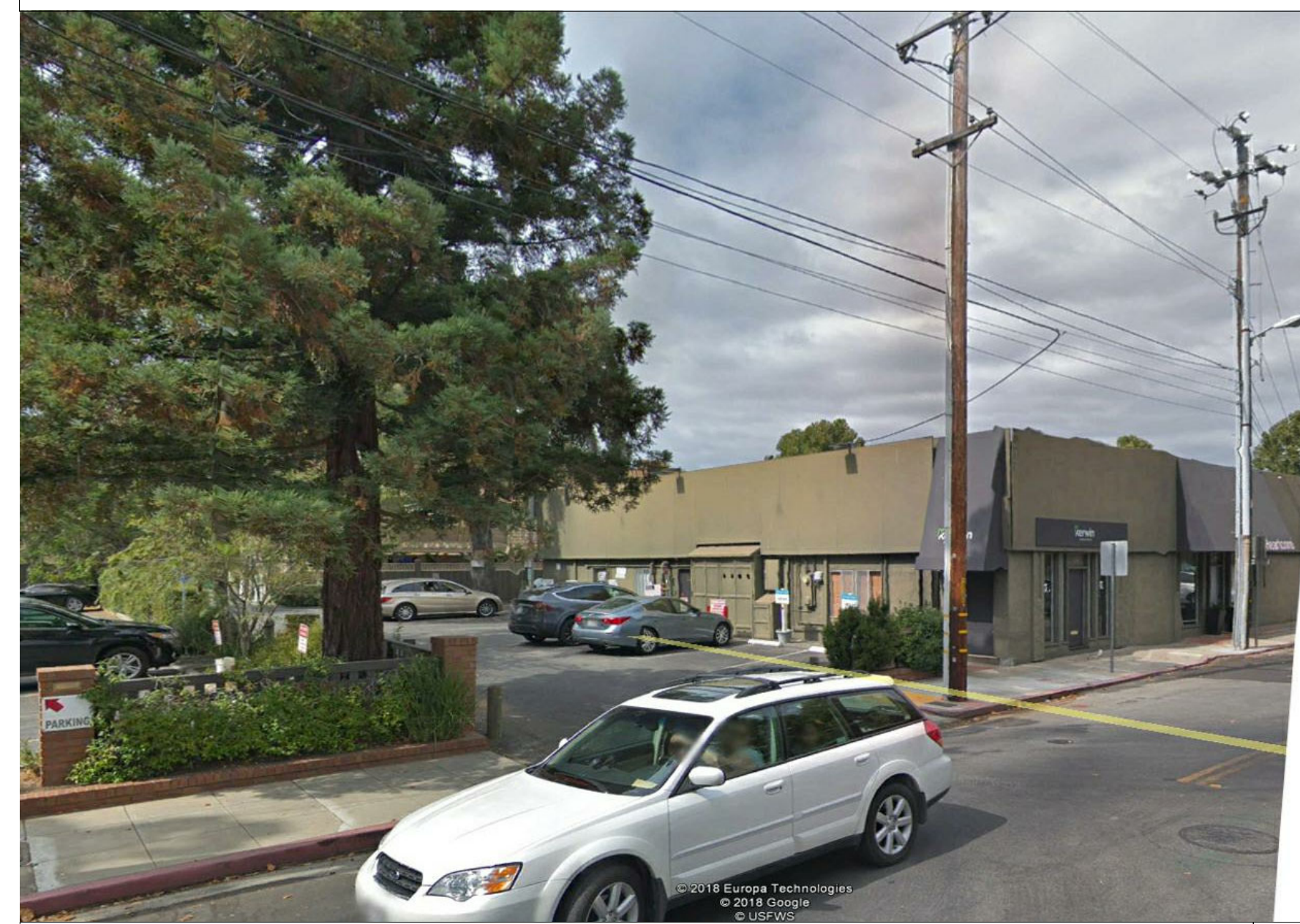
PG&E UTILITIES AND AT&T CABLE BEHIND EXISTING BUILDING 3.
