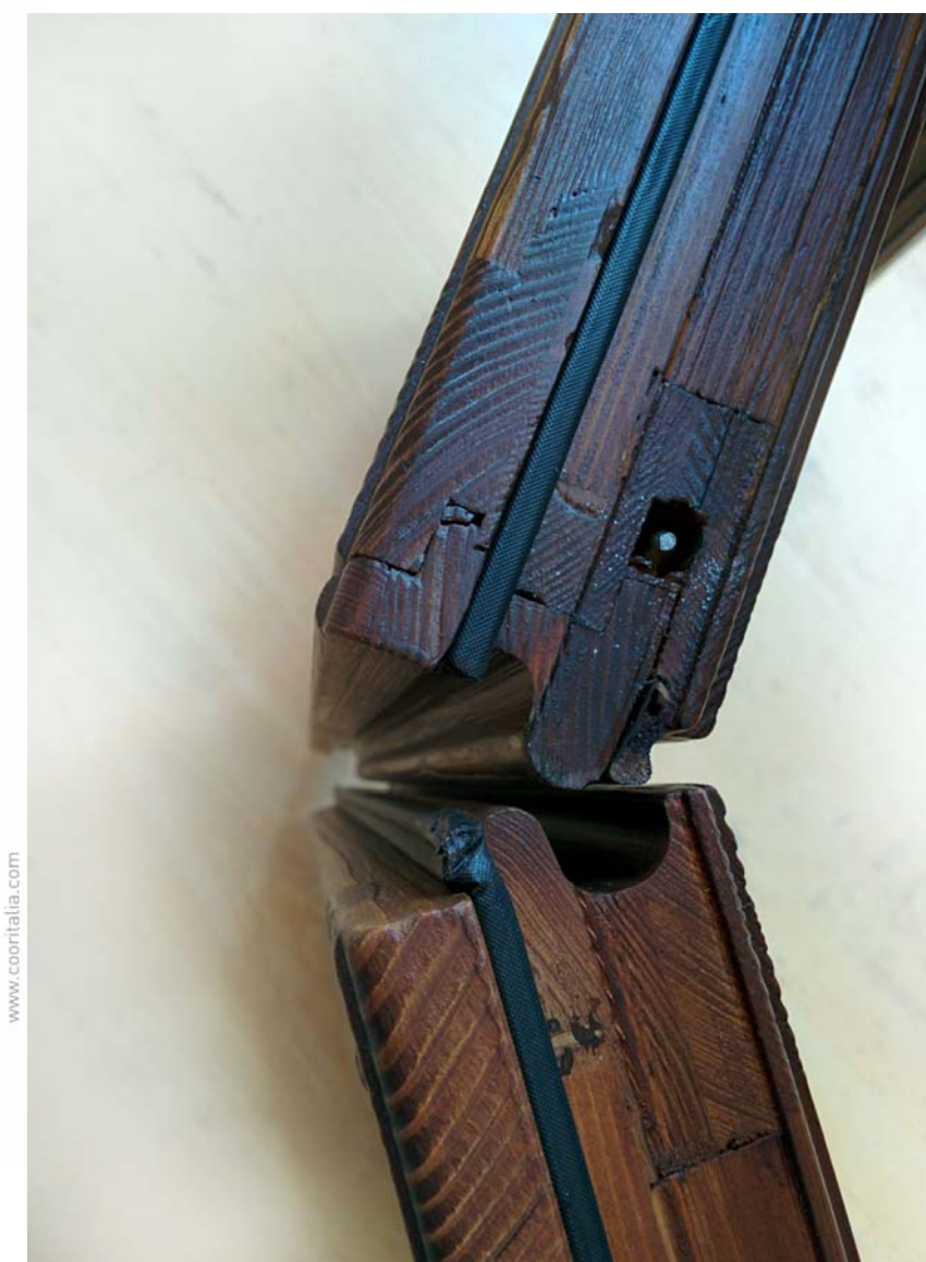
TOP VIEW OF CASEMENT COMING TOGETHER
