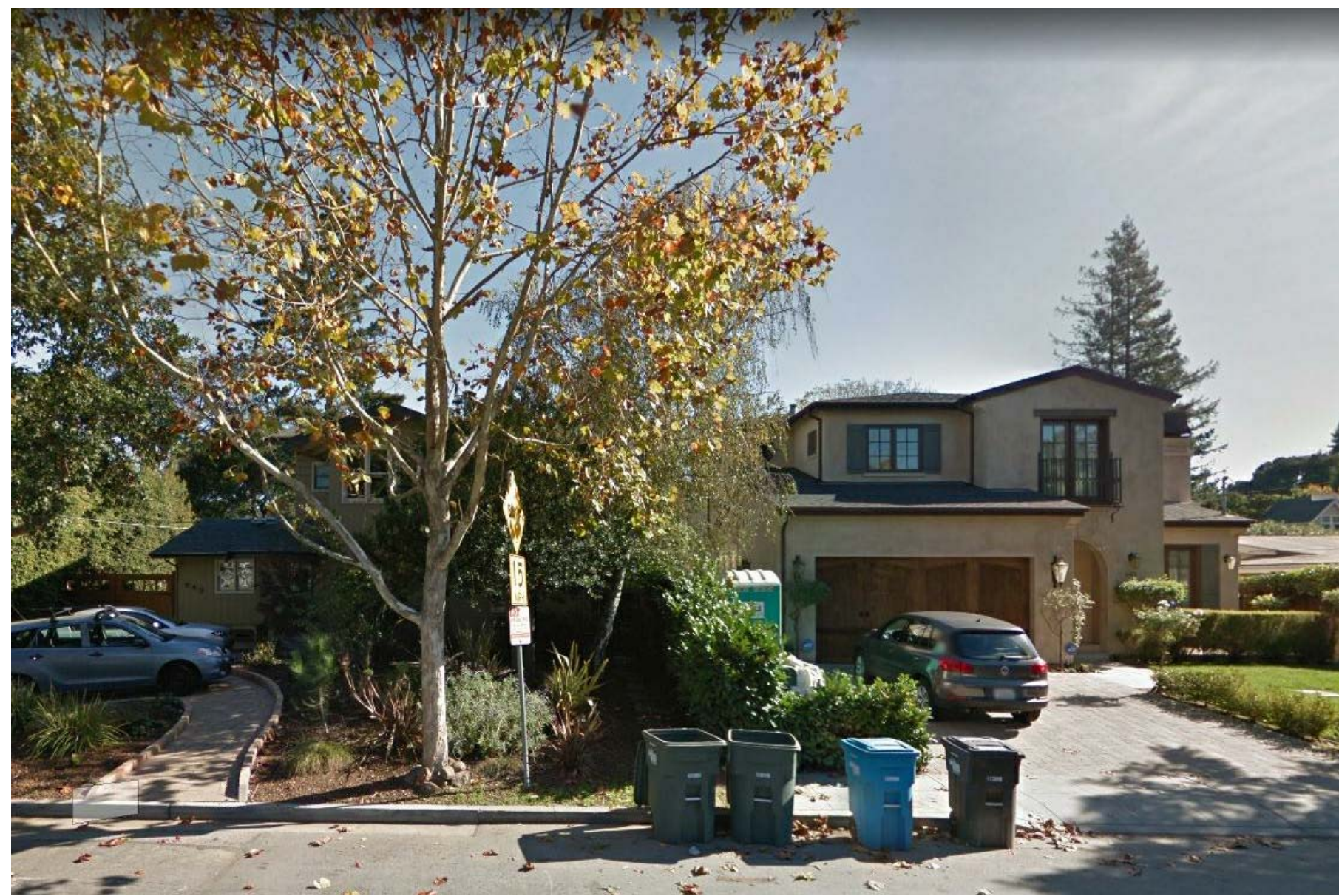
EXISTING NEIGHBORHOOD HOUSE - 649/ 665 CAMBRIDGE 8.
