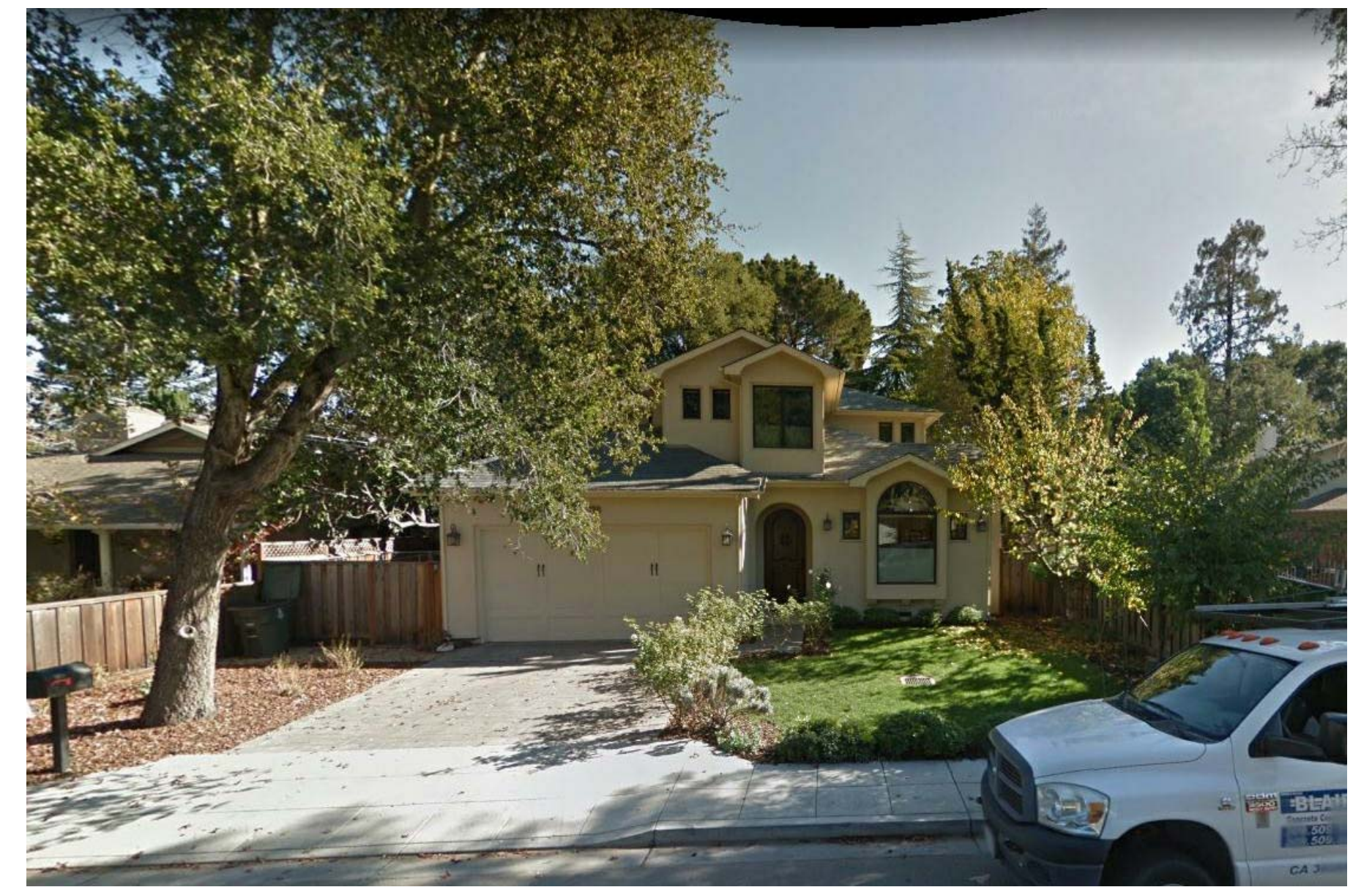
EXISTING NEIGHBORHOOD HOUSE - 739 CAMBRIDGE 2.
