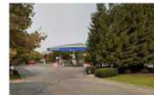
CANOPY LOOKING NORTH
