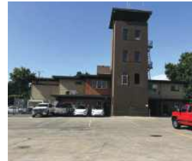
EXISTING MENLO PARK FIRE STATION NO. 01 TO BE DEMOLISHED - ELEVATION (REAR)
