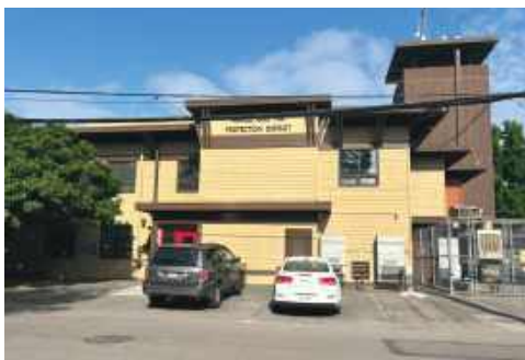
EXISTING MENLO PARK FIRE STATION NO. 01 TO BE DEMOLISHED - SANTA MONICA ROAD ELEVATION (EAST SIDE)
