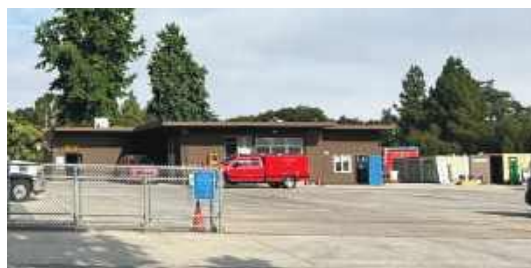
EXISTING MENLO PARK MAINTENANCE BLDG TO BE DEMOLISHED - SANTA MONICA ROAD ELEVATION (EAST SIDE)
