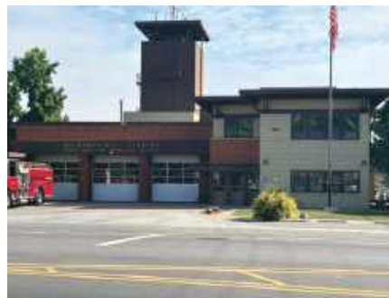
EXISTING MENLO PARK FIRE STATION NO. 01 TO BE DEMOLISHED - MIDDLEFIELD ROAD ELEVATION (FRONT)
