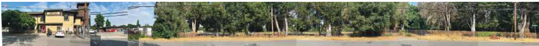
EXISTING MENLO PARK FIRE STATION NO. 01 & MAINTENANCE BUILDING TO BE DEMOLISHED - SANTA MONICA ROAD ELEVATION (EAST SIDE)
