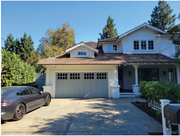
EXISTING VIEW FROM END OF DRIVEWAY
