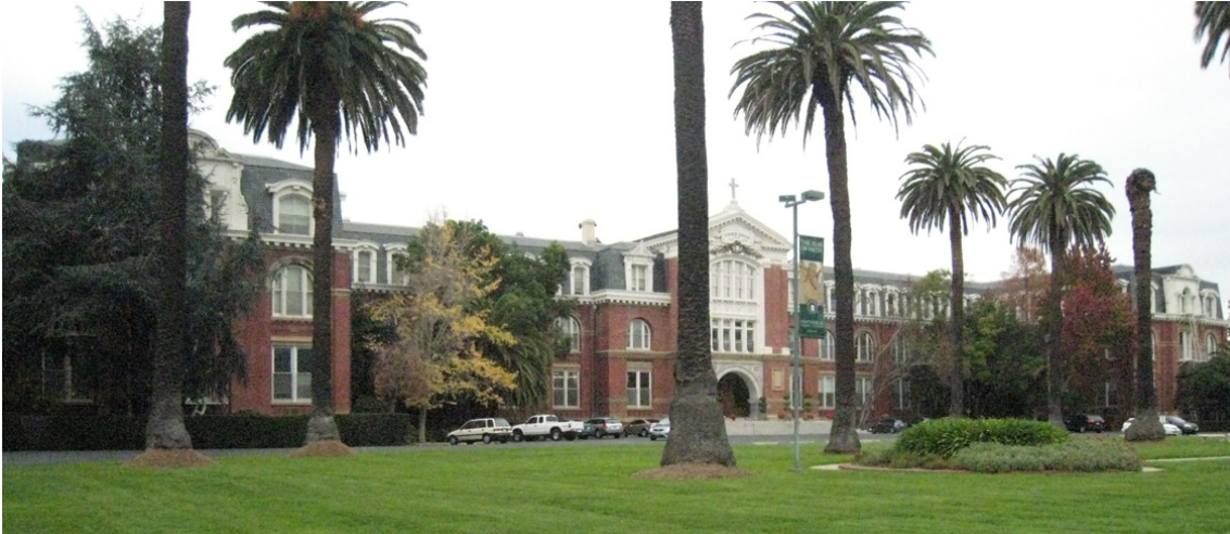
View 3: View of the administration wing of the seminary looking across the elliptical lawn.
