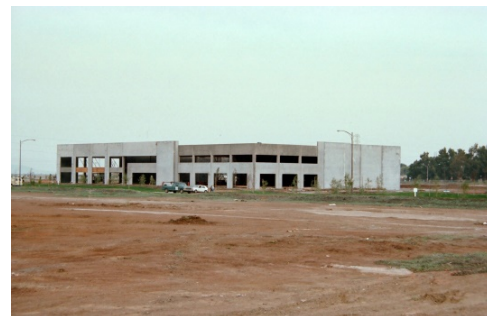
Office construction in the 1980s
