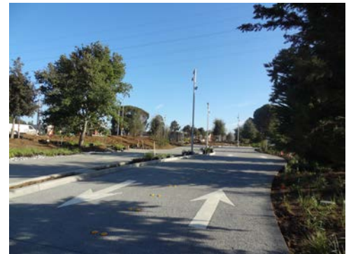
Walking and biking route under Bayfront Expressway
