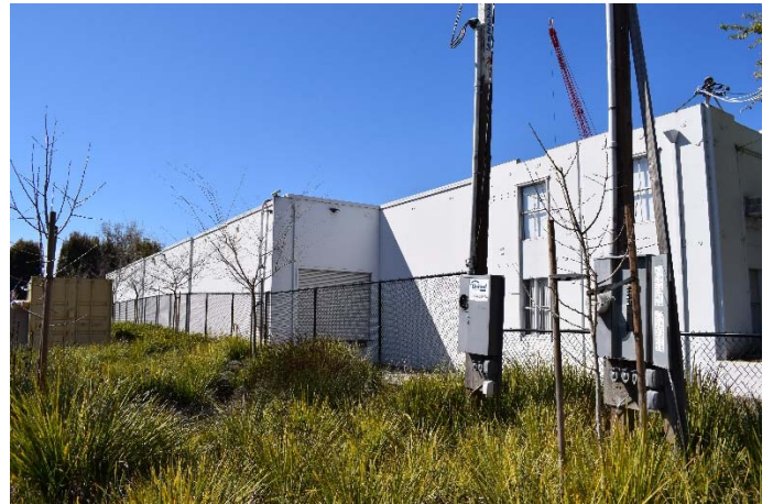
Figure 3. View of east façade, facing southwest, 3/6/2018.
