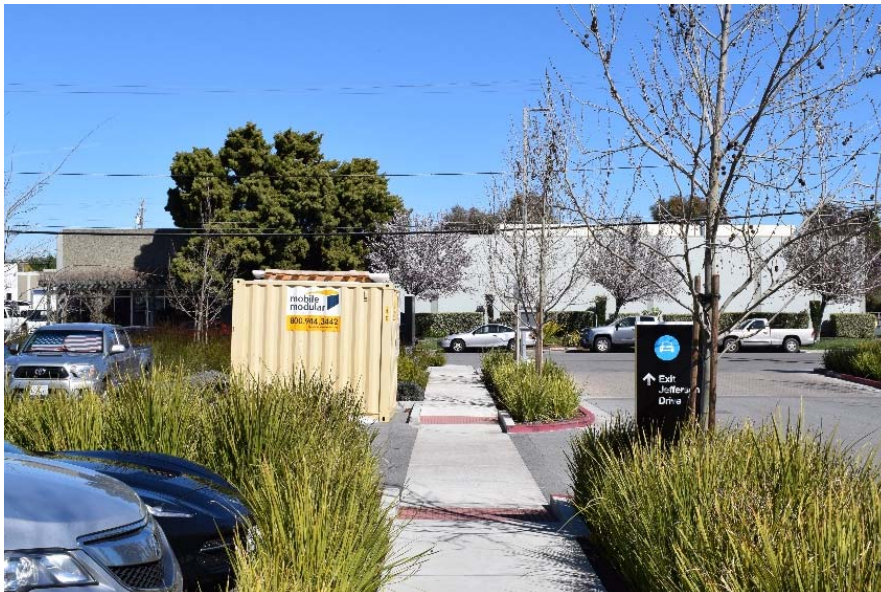
Figure 1: View of South (primary) façade, facing north. Source: ICF.
