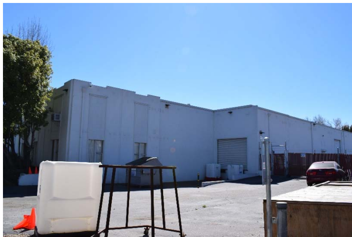
Figure 4. View of west facade, facing southeast, 3/6/2018.
