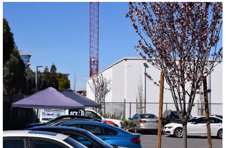
Figure 5. View of south (rear) and east façades, facing west, 3/6/2018.
