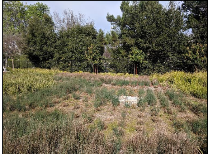
Photo 2. Bioretention basin located on the eastern edge of the project site.
