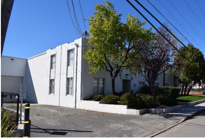
Figure 2. View of north (primary) and east facades, facing southwest, 3/6/2018.
