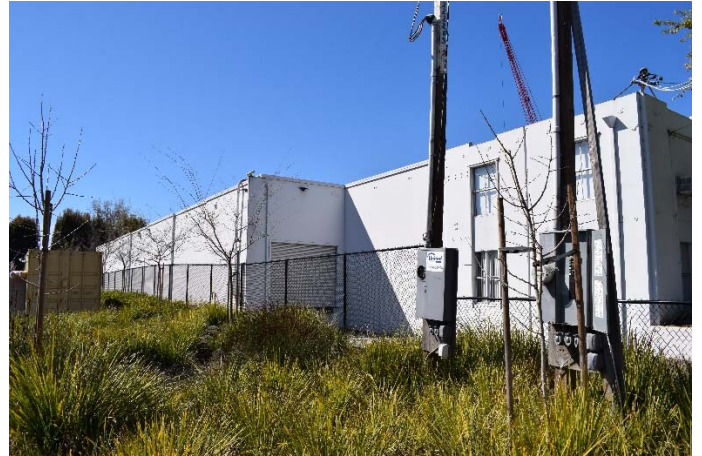
Figure 3. View of east façade, facing southwest, 3/6/2018.
