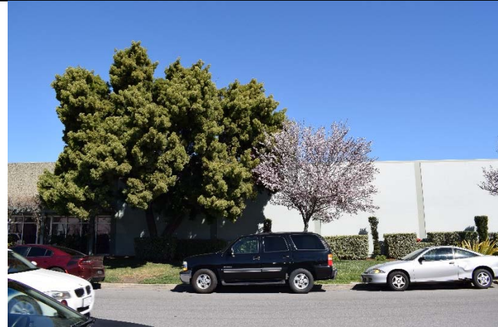
Figure 2. View of south (primary) façade, facing north, 3/6/2018.
