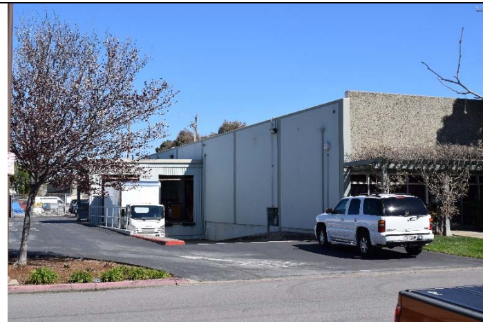
Figure 4. View of west façade, facing northeast, 3/6/2018.
