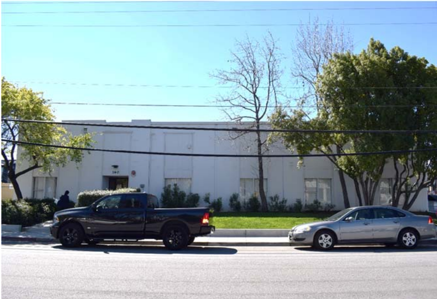
Figure 1: View of North (primary) façade, facing south. Source: ICF.
