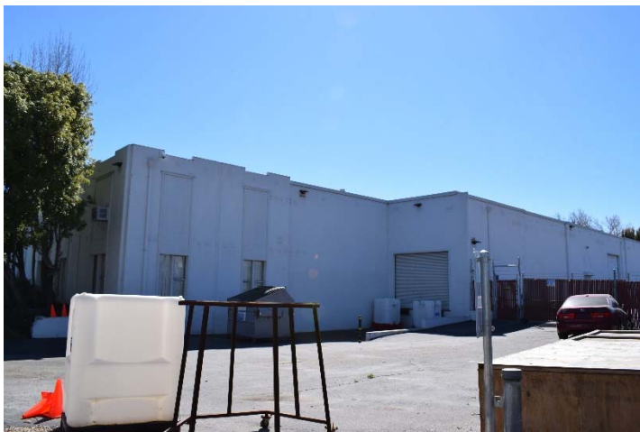
Figure 4. View of west facade, facing southeast, 3/6/2018.
