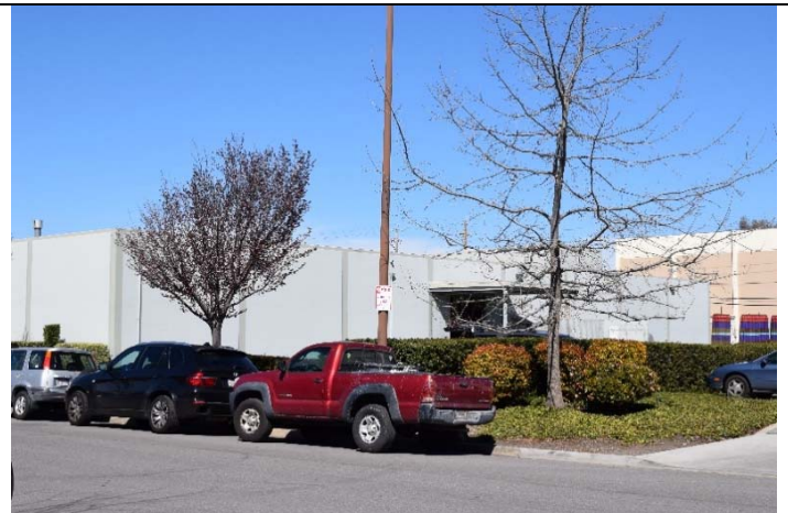
Figure 5. Detail view of east façade facing northwest, 3/6/2018.
