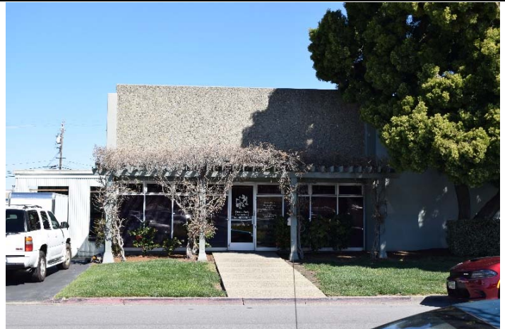
Figure 3. Detail view of south façade facing north, 3/6/2018.
