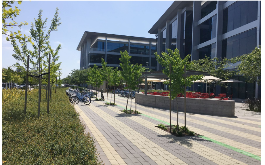
B. View of Buildings 1 and 2 Facing East.
