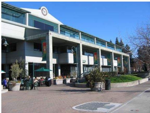
Existing 3-story retail / office space along El Camino Real (Menlo Park, California)
