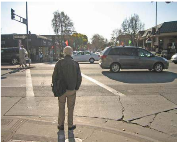
Poor accessibility and linkages between key spaces (Menlo Park, California)
