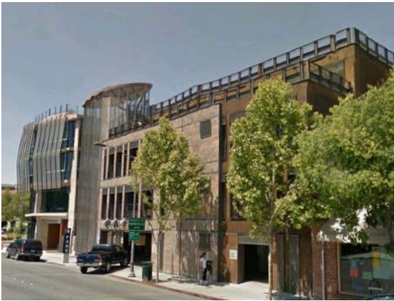
Guideline E.3.7.10. Parking garage successfully avoiding a monolithic massing by change in height, material, pattern and color (Palo Alto, California)
