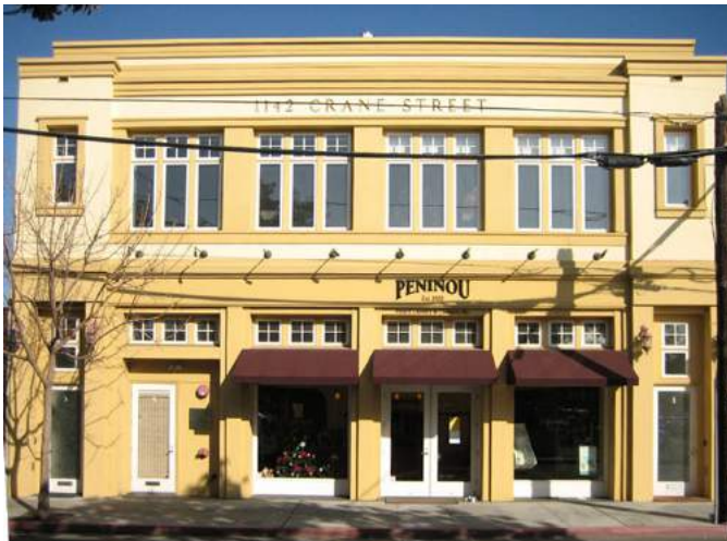
Guideline E.3.5.19. Storefront elements lend visual interest to facades (Menlo Park, California)
