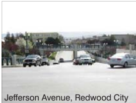
Jefferson Avenue, Redwood City Underpass crossing in Redwood City (depressed roadway)
