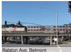
Ralston Ave, Belmont Ralston Ave, Belmont Underpass crossing in Belmont (raised rail line with depressed roadway)
