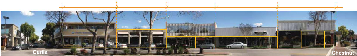
Downtown exhibits a pattern of smaller buildings and storefronts as compared to buildings on much of El Camino Real.
