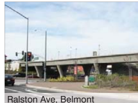
Ralston Ave, Belmont Ralston Ave, Belmont Underpass crossing in Belmont (raised rail line with depressed roadway)
