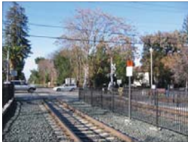
At-grade crossing at Oak Grove Avenue, Menlo Park
