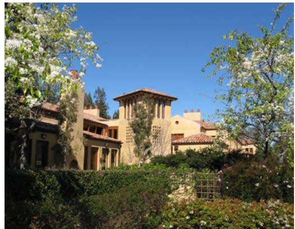
Existing office space at 1600 El Camino Real (Menlo Park, California)
