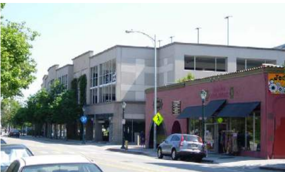
Guideline E.3.7.12. Overall building façade compatible with surrounding building character (Santa Cruz, California)
