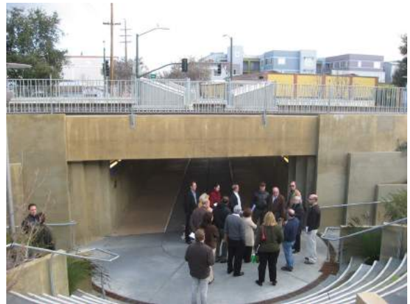
Pedestrian/bicycle tunnel linkage (Palo Alto, California)
