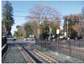
At-grade crossing at Oak Grove Avenue, Menlo Park
