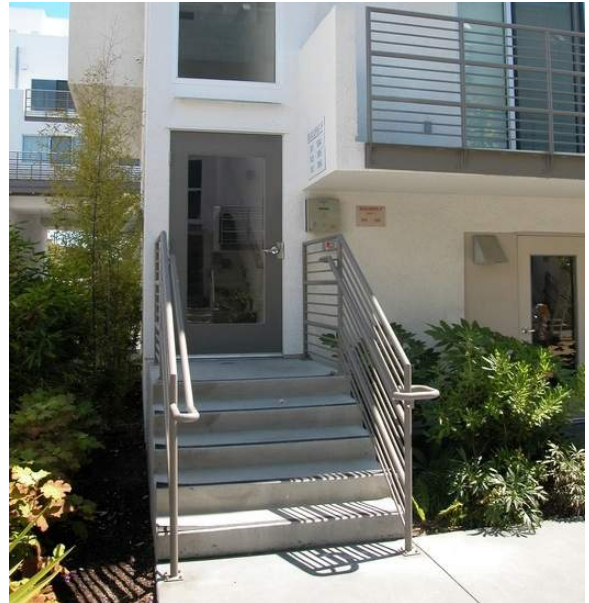
Guideline E.3.5.12. Ground floor residential units encouraged to have their entrance from the street
