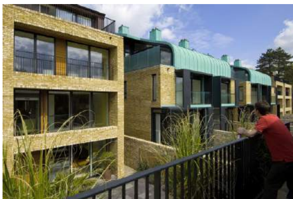
Guideline E.3.6.05. Private open space as an extension of the indoor living area (Cambridge, England)
