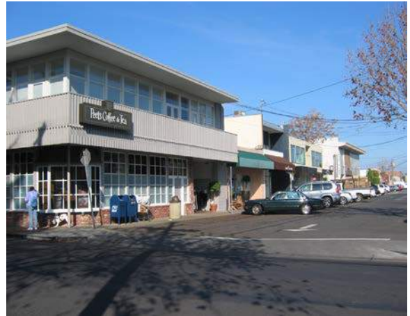
Peet's Coffee at the corner of Santa Cruz Avenue and University Drive (Menlo Park, California)
