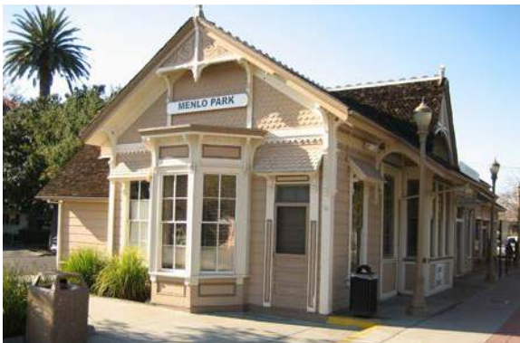
Caltrain Station is a local landmark (Menlo Park, California)
