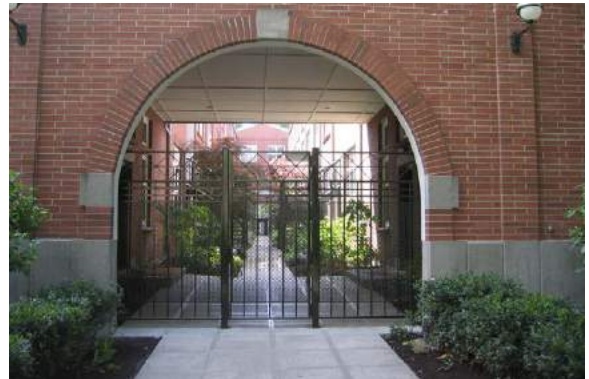
Guideline E.3.5.09. Inviting, prominent shared entry from a central courtyard facing the street (Portland, Oregon)
