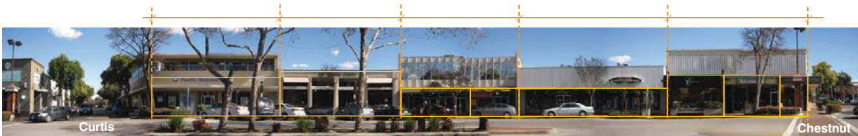
Downtown exhibits a pattern of smaller buildings and storefronts as compared to buildings on much of El Camino Real.
