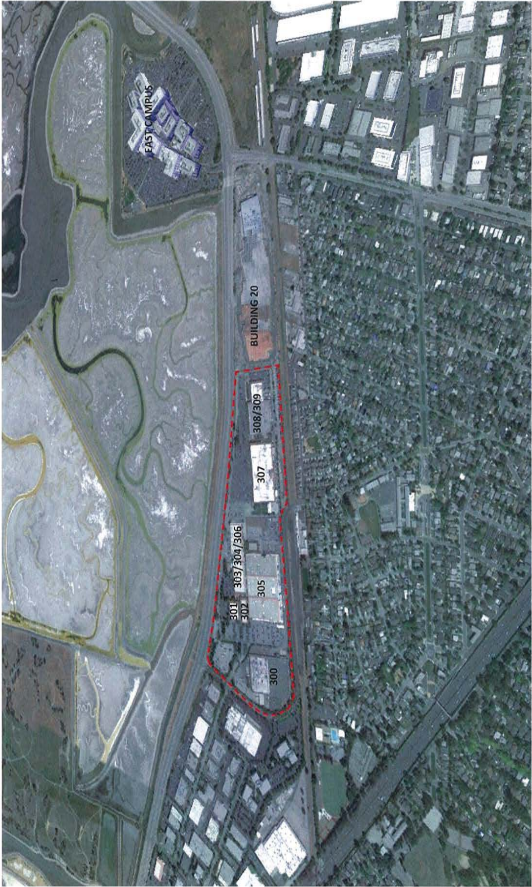
AERIAL SITE VIEW LOOKING NORTH
