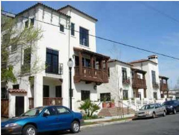
✔ Yes: Varied building mass and height with appropriate façade articulation promotes visual interest (Mountain View, California)
