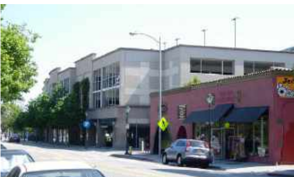
Guideline E.3.7.12. Overall building façade compatible with surrounding building character (Santa Cruz, California)
