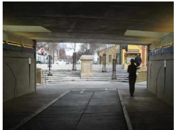
Grade separated pedestrian/bicycle linkage (Palo Alto, California)
