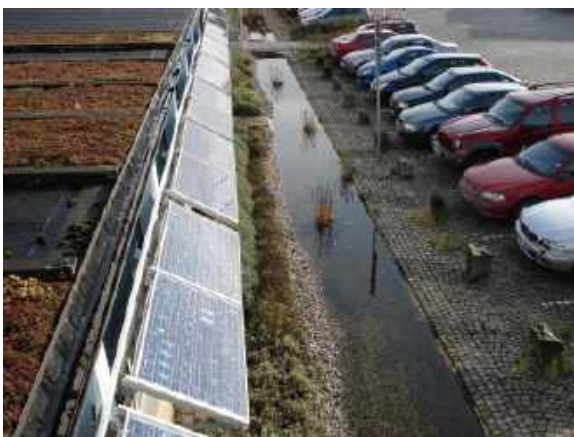
Parking plaza designed according to sustainable practices such as augmenting the permeability of surfaces, mitigating heat island effect and producing renewable energy (Malmo, Sweden)
