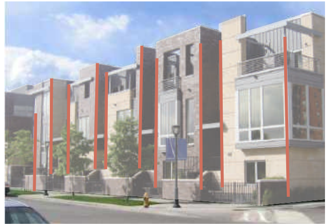
Building façade modulation
