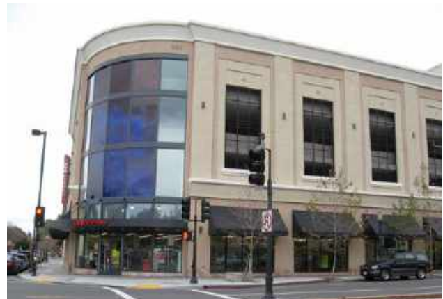
Public parking garage wrapped with retail use (Mountain View, California)
