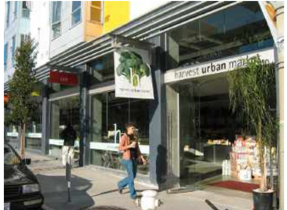
Standard E.3.5.02 Well designed, transparent ground floor treatment ensuring a pleasant and safe pedestrian experience (San Francisco, California)
