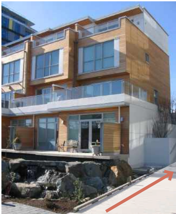
Building break (Victoria, British Columbia)
