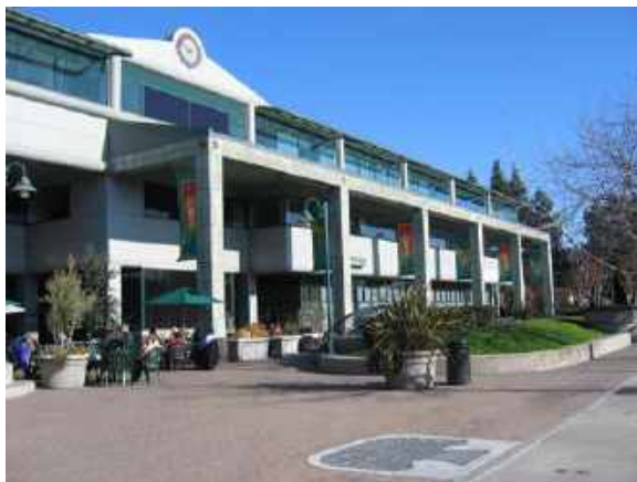
Existing 3-story retail / office space along El Camino Real (Menlo Park, California)
