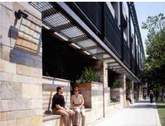
Guideline E.3.7.11. Screening of parking garage with seating areas and landscaping (Sacramento, California)
