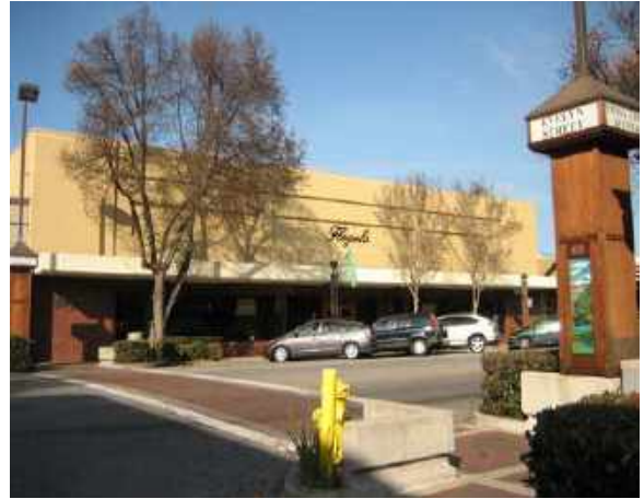
Flegel's Home Furnishings, a major independent retailer located downtown at the corner of Santa Cruz Avenue and Evelyn Street (Menlo Park, California)
