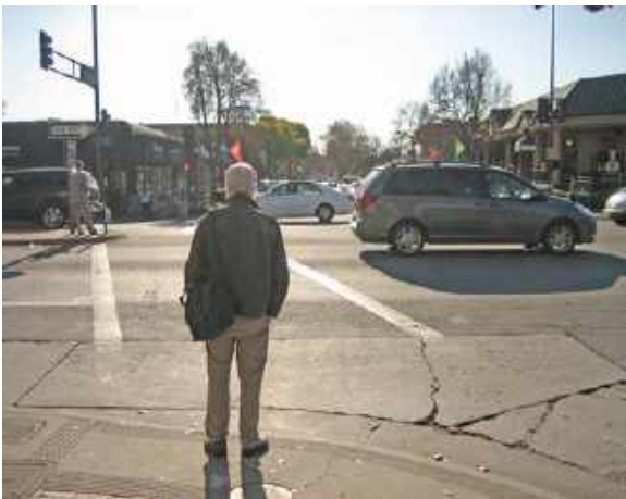
Poor accessibility and linkages between key spaces (Menlo Park, California)
