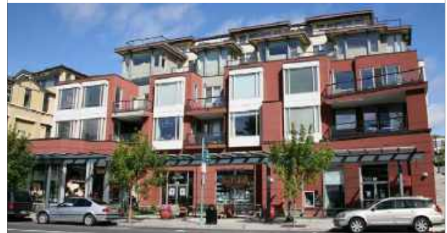
✓ Yes: Varied primary building façade plane (Kirkland, Washington)
