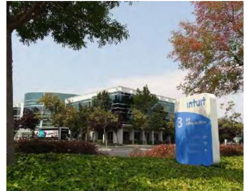
Development of tech firm offices continue today
