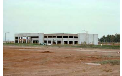
Office construction in the 1980s
