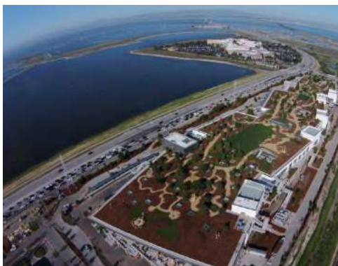
Facebook Building 20 and East Campus
