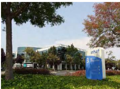
Offices originally constructed for Intuit
