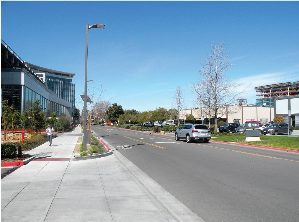
Photo 5: Existing buildings south of the project site, as seen from Independence Drive, south of the project site.
