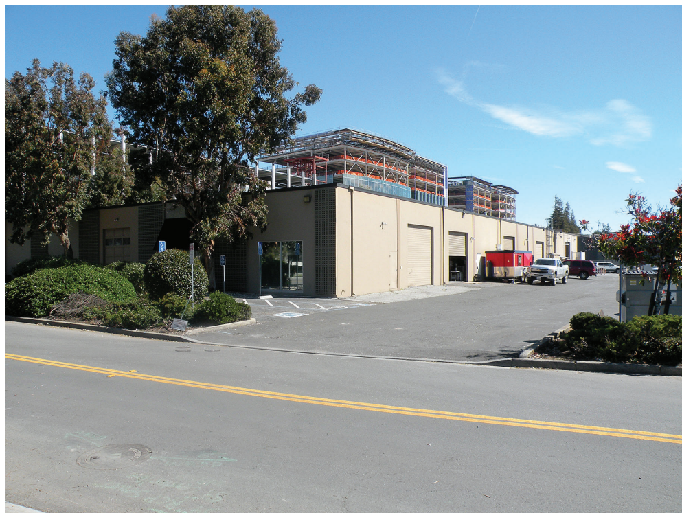
Photo 2: Existing building at 104 Constitution Drive, as seen from Independence Drive
