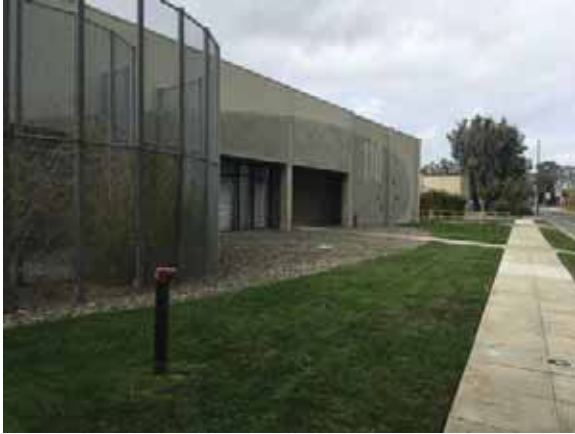
Photo 1. The project site consists of commercial buildings surrounded by hardscape with narrow, interrupted areas of landscaping.
