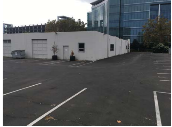
Photo 2. The project site consists of commercial buildings surrounded by hardscape with narrow, interrupted areas of landscaping.
