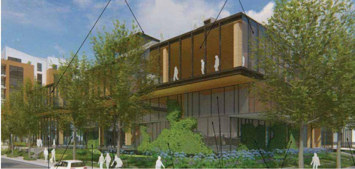
Figure 4. The predominantly glazed facades of the office building increase the probability that birds will collide with these facades.
