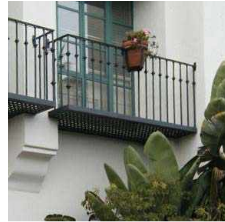
12. Metal Guardrail and Railing
