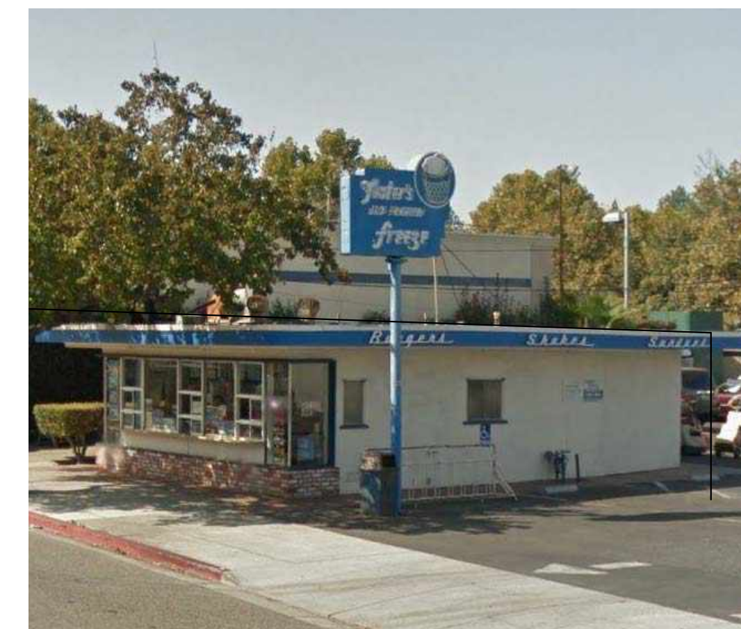
2 (E) Struct. A - R. Side East Elevation A4.10 1/8" = 1'-0" (E) STRUCT. A - L. SIDE WEST ELEVATION SIMILAR
