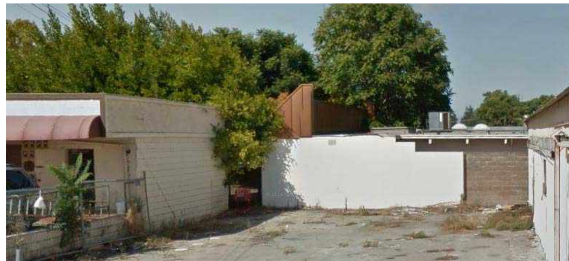
2 (E) Struct. G - R. Side South Elevation A4.11 1/8" = 1'-0" (E) STRUCT. G - L. SIDE NORTH ELEVATION SIMILAR
