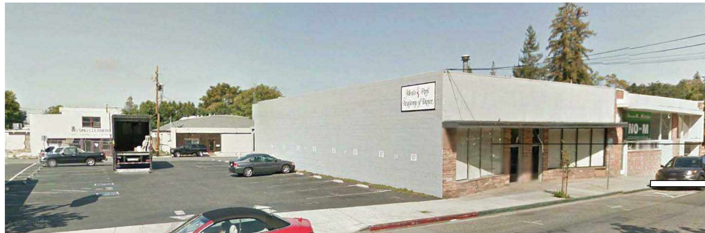
6 (E) Struct. B - L. Side West Elevation A4.10 1/8" = 1'-0" (E) STRUCT. C - R. SIDE EAST ELEVATION SIMILAR
