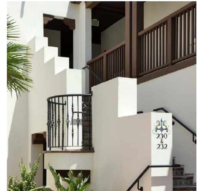
14. Wooden Posts at Balconies and Trellises
