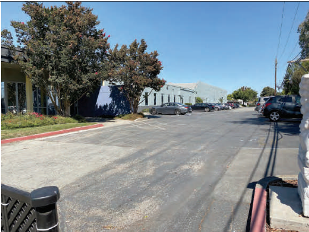
Photo 1: Existing building at 141 Jefferson Drive, as seen from Jefferson Drive
