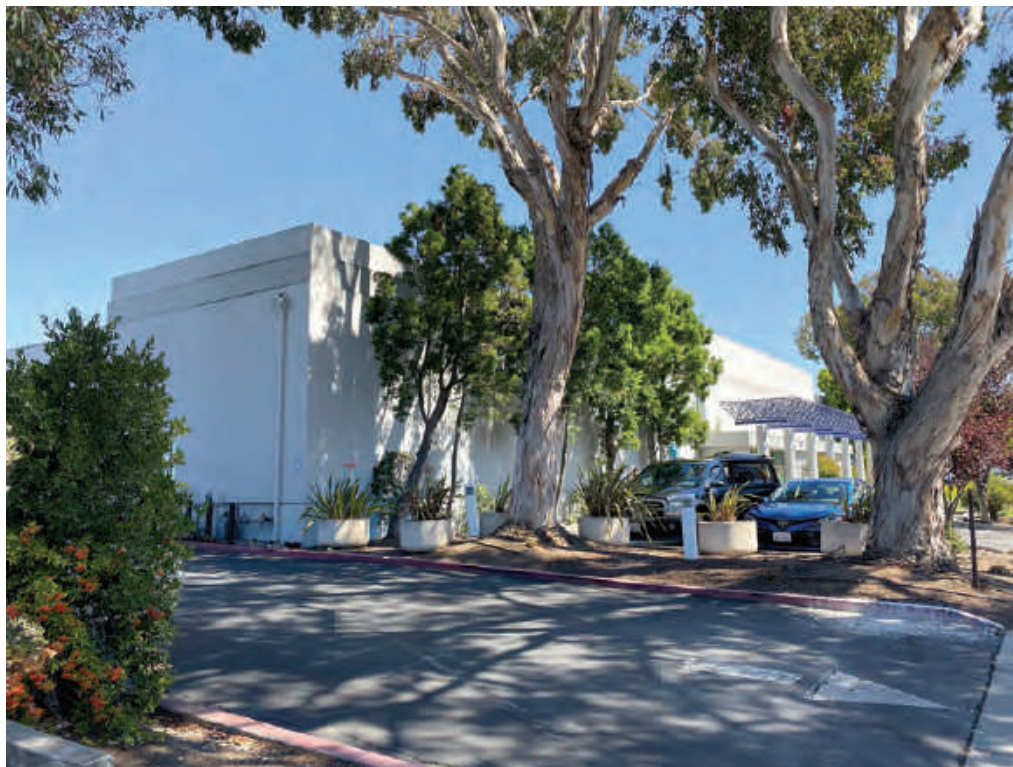
Photo 4: Existing building east of the project site (Synergy Badminton Club), as seen from Jefferson Drive
