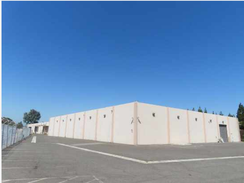
Exhibit 6. Main (south) and east elevation. View looking northwest (IMG_0860).
