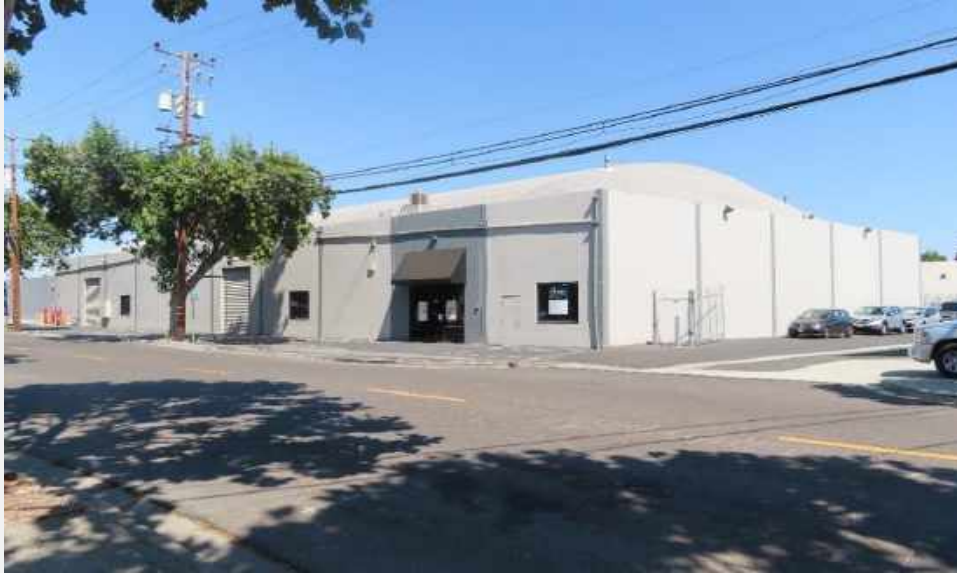
Exhibit 1. Overview of 985 O'Brien Drive showing main elevation (south) and east elevation. View looking northwest (IMG_0842).
