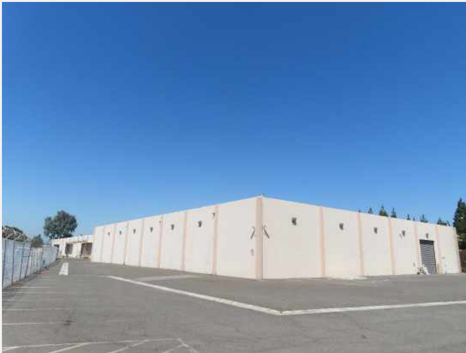
Photograph 6. Main (south) and east elevation. View looking northwest (IMG_0860).
