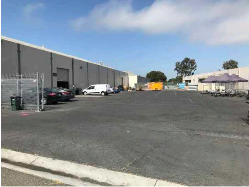
Photograph 1: Back lot at 985 O'Brien Drive.
