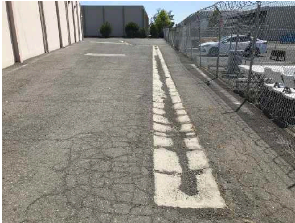
Photograph 10: Stormwater trench outside building at 1320 Willow Road.
