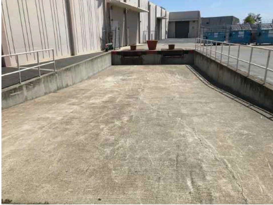
Photograph 11: Loading dock at 1320 Willow Road.
