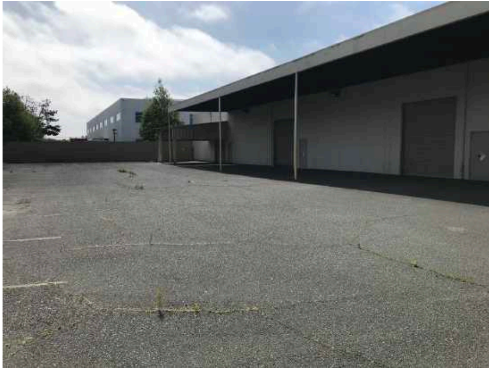
Photograph 7: Back lot at 1001 O'Brien Drive.
