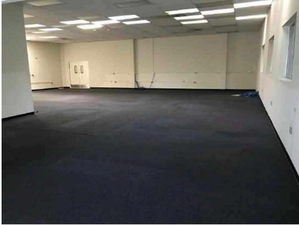
Photograph 9: Office area in building at 1001 O'Brien Drive.
