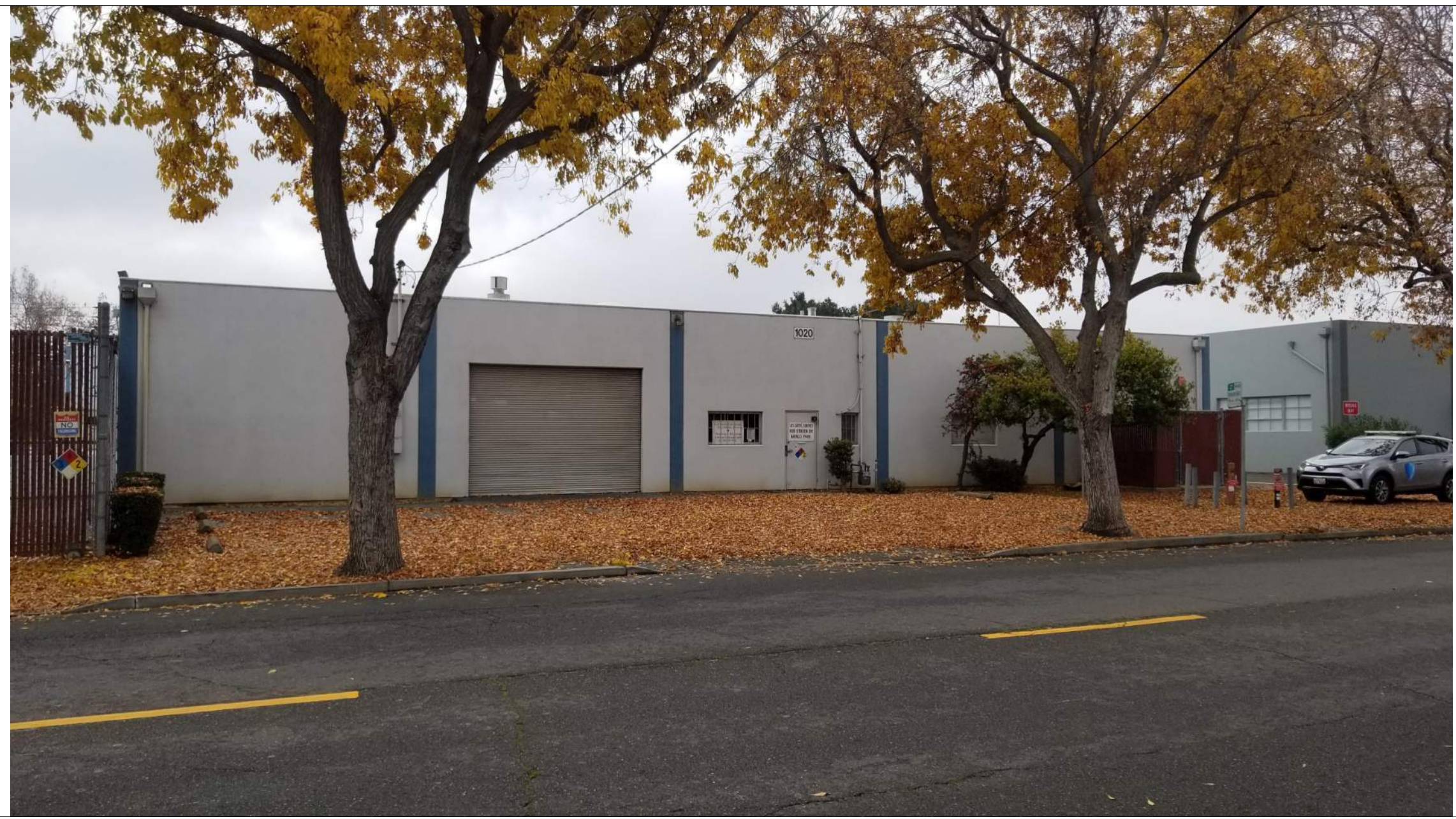
3 1020 O'BRIEN (TO BE DEMOLISHED)
