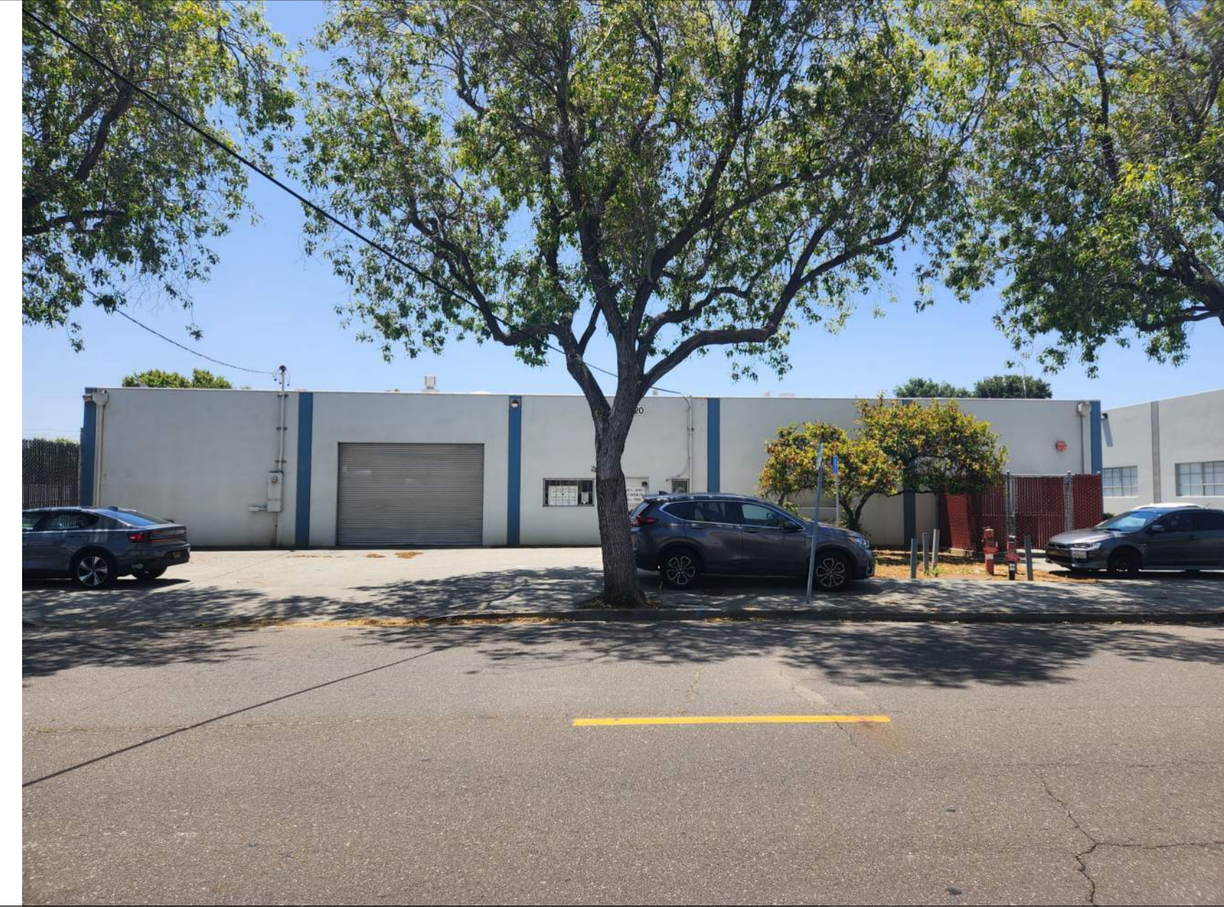
1 1020 O'BRIEN - NORTH (TO BE DEMOLISHED)
