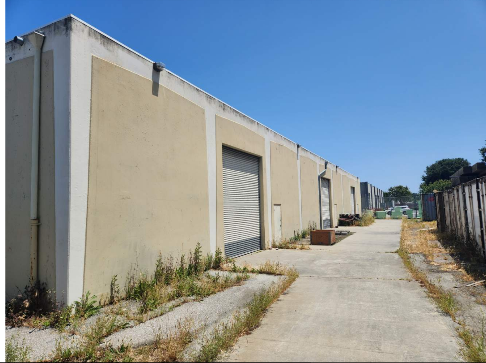
9 1030 O'BRIEN - SOUTH (TO BE DEMOLISHED)
