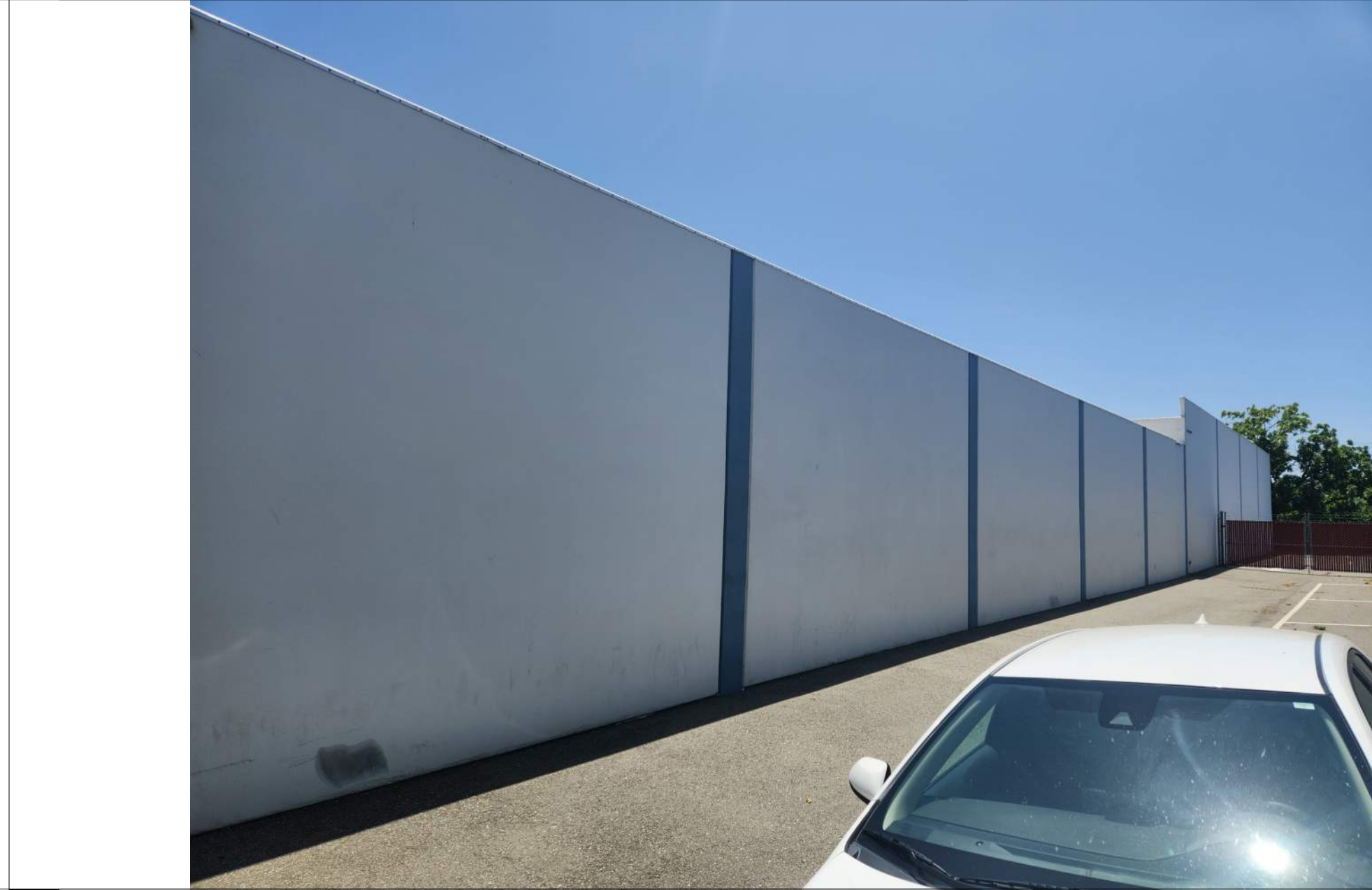
5 1020 O'BRIEN - WEST (TO BE DEMOLISHED)
