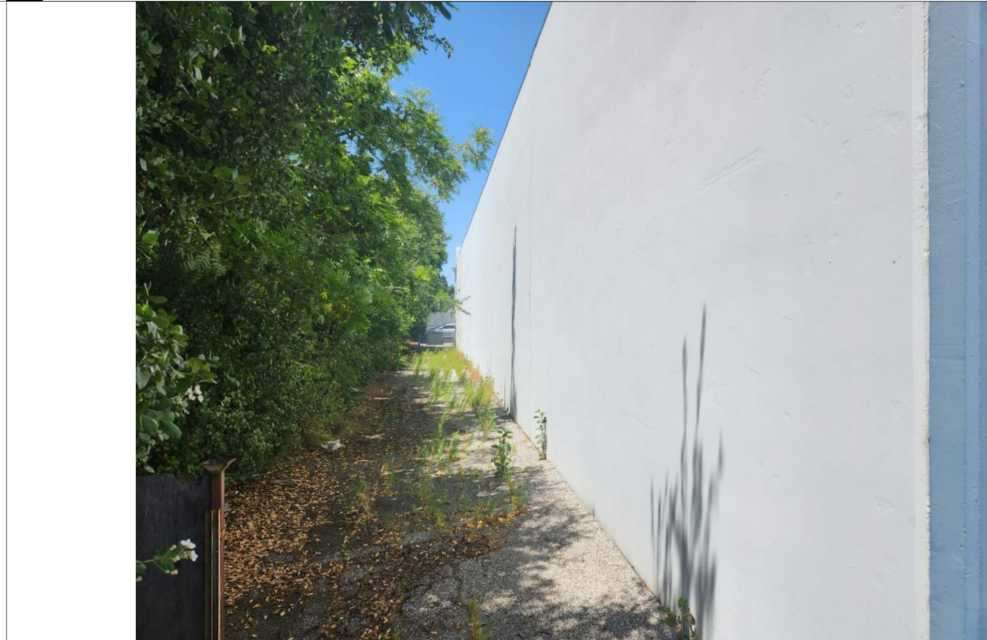
4 1020 O'BRIEN - SOUTH (TO BE DEMOLISHED)
