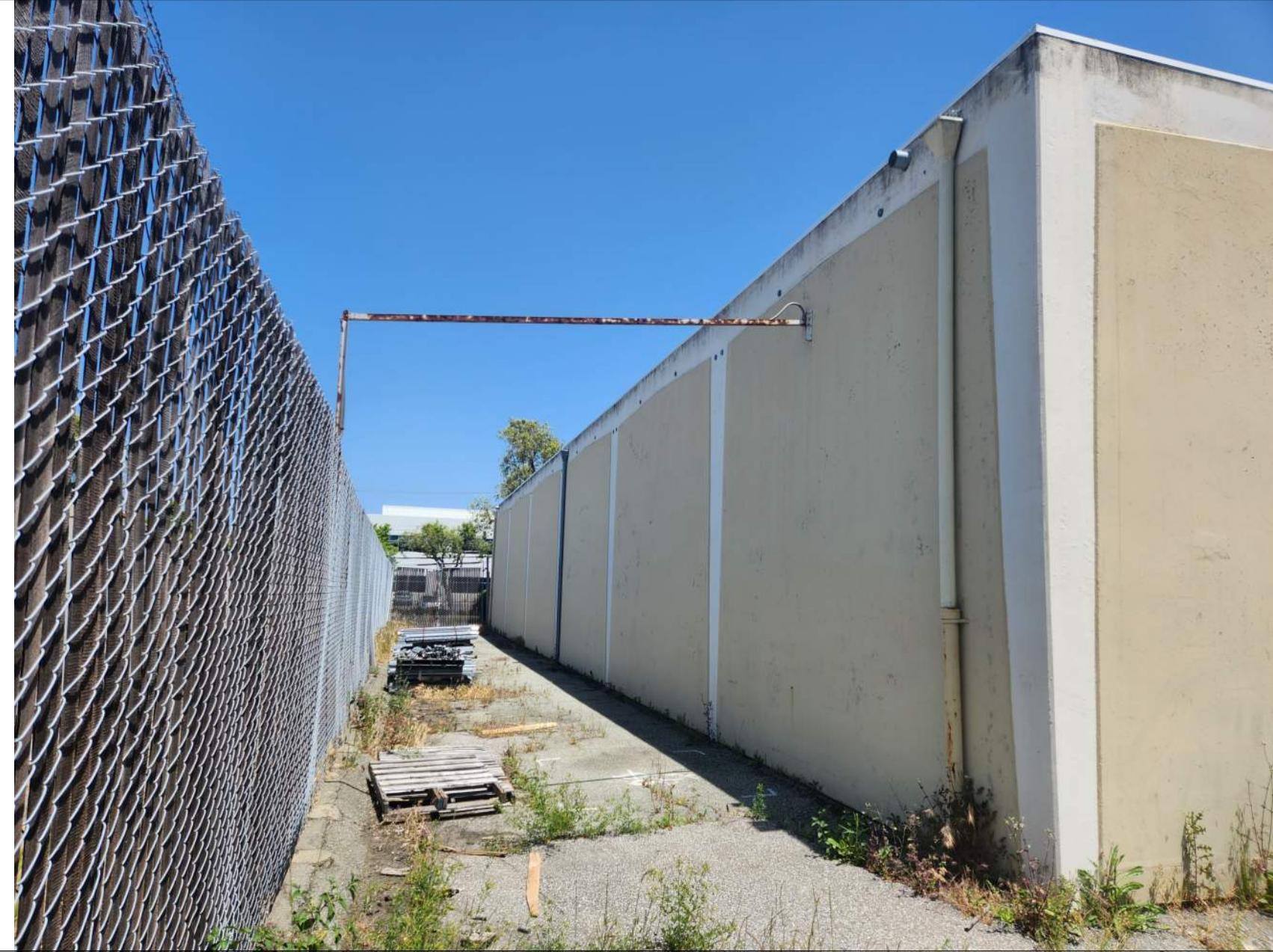
10 1030 O'BRIEN - WEST (TO BE DEMOLISHED)
