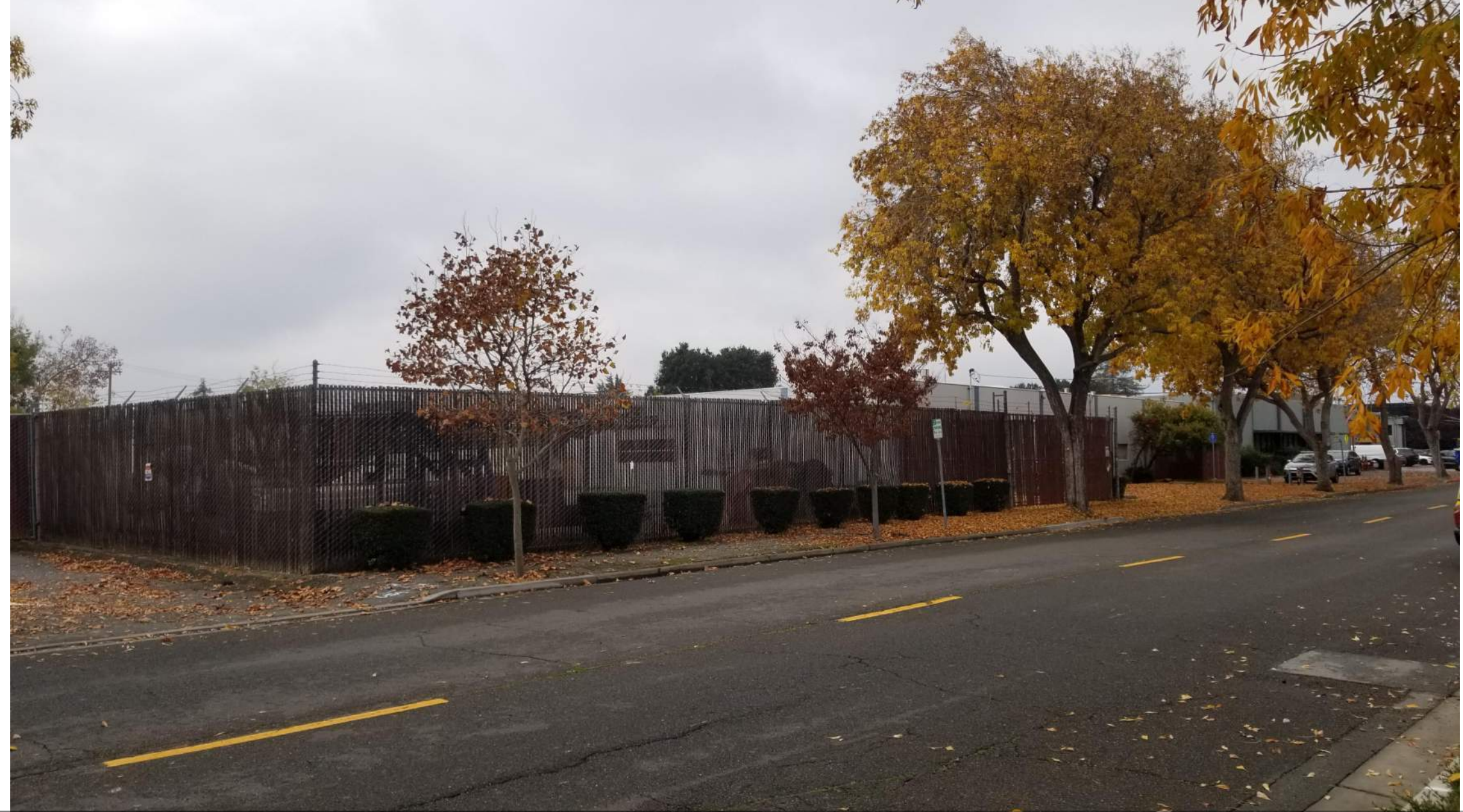
2 1020 O'BRIEN (TO BE DEMOLISHED)
