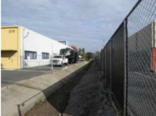
View of Drainage Channel (Parcel 35)
