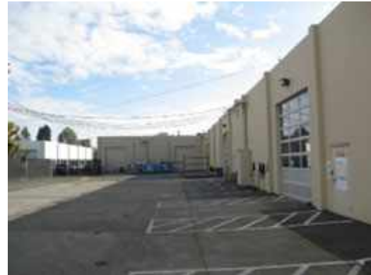
Rear Elevation of 1125 O'Brien Drive
