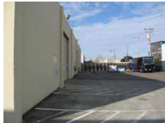
Rear Elevation of 1105 O'Brien Drive
