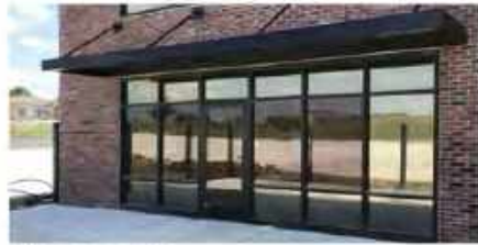
W2 STOREFRONT ALUMINIUM STOREFRONT BLACK FRAME FINISH
