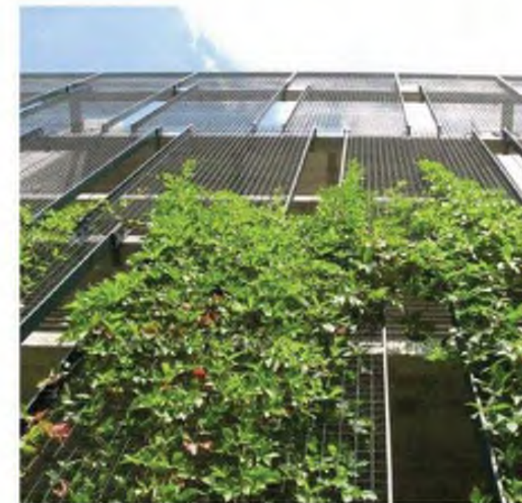
F1 GREEN SCREEN STEEL FRAMED PANEL WITH STEEL WIRE GRIDS 24X 4' WIDE PANELS SPACED WITH 4" GAPS HORIZONTALLY
