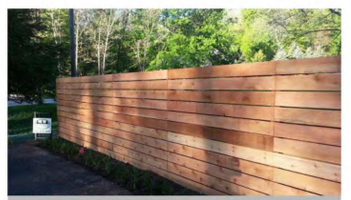
PERIMETER FENCE 72" TALL HORIZONTAL WOOD PLANKS
