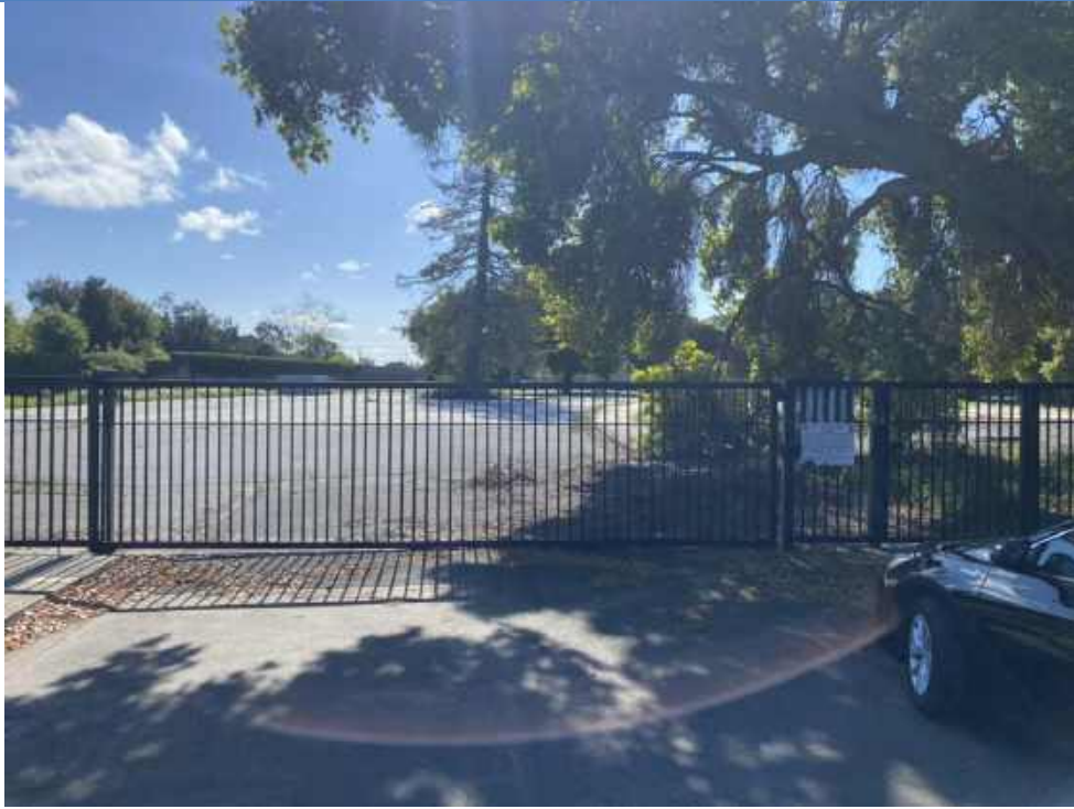
PHOTO 1: View of the entrance of the Site along Sheridan Drive, looking southeast.
