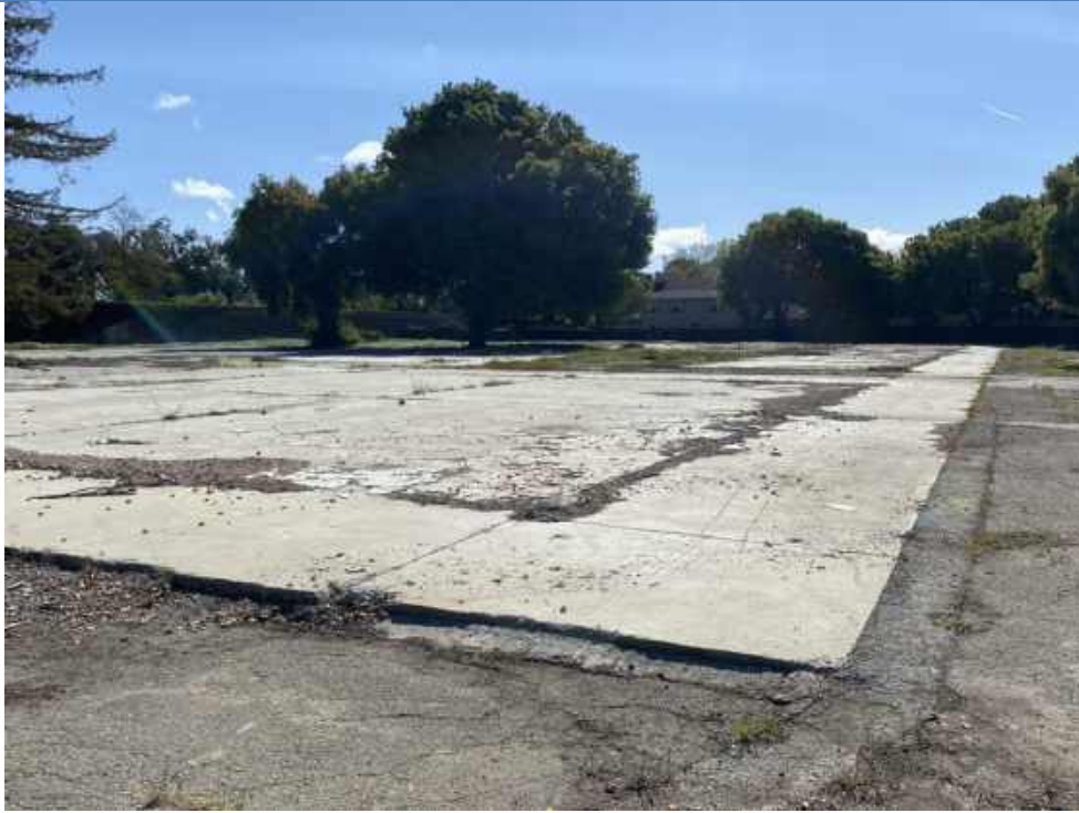
PHOTO 9: View of large remnant concrete building floor slabs in the southwestern portion of the Site, looking southeast.
