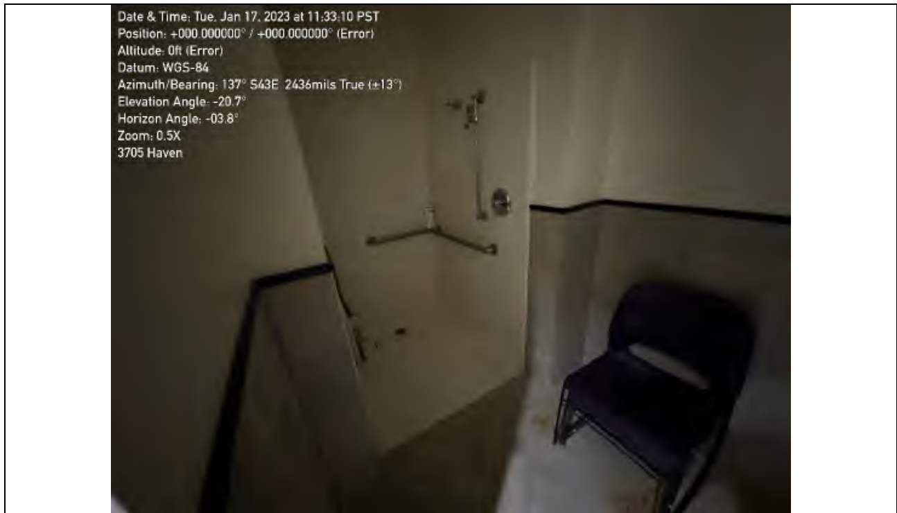
Photo #11 View of shower with floor drain in men's bathroom.
