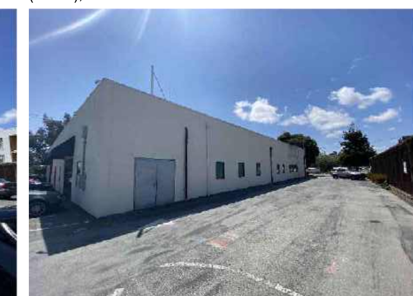
8. VIEW FROM NW PORTION LOOKING SW
