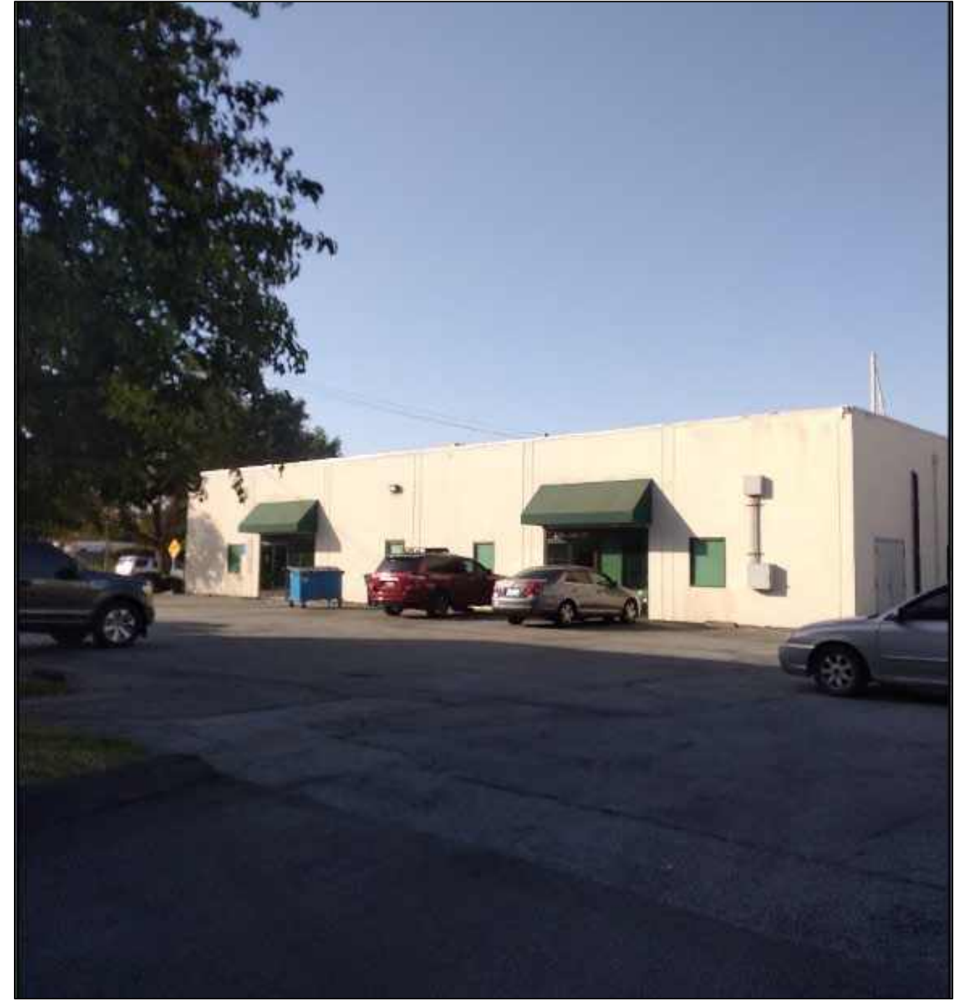
Photograph 4. West side of parcel facing the existing building.
