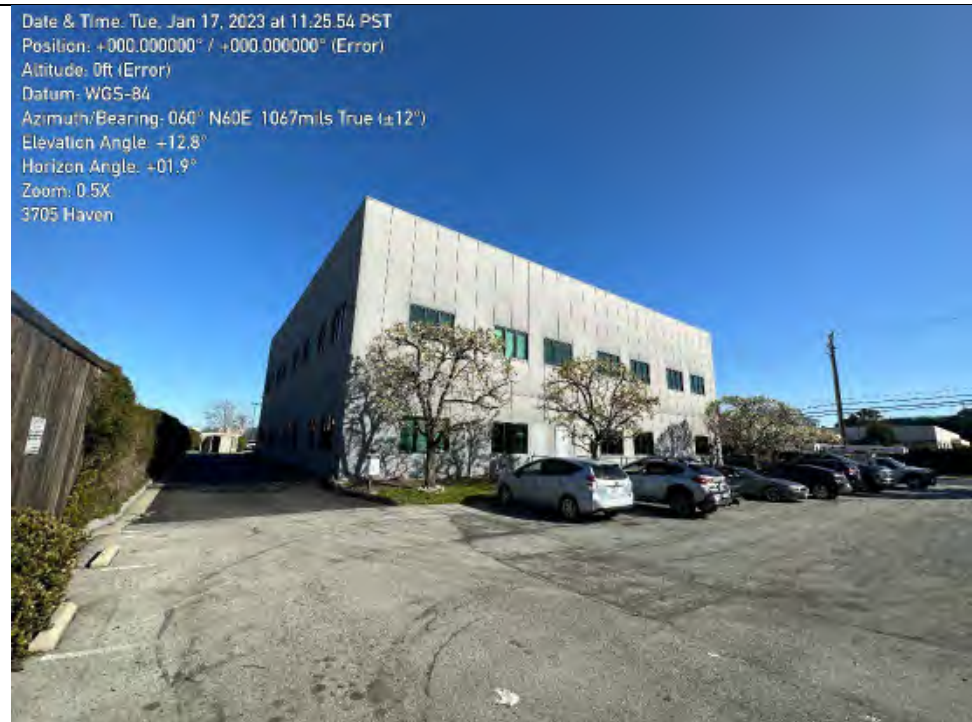
Photo #16 View of commercial development on the adjacent site to the north of the Property.
