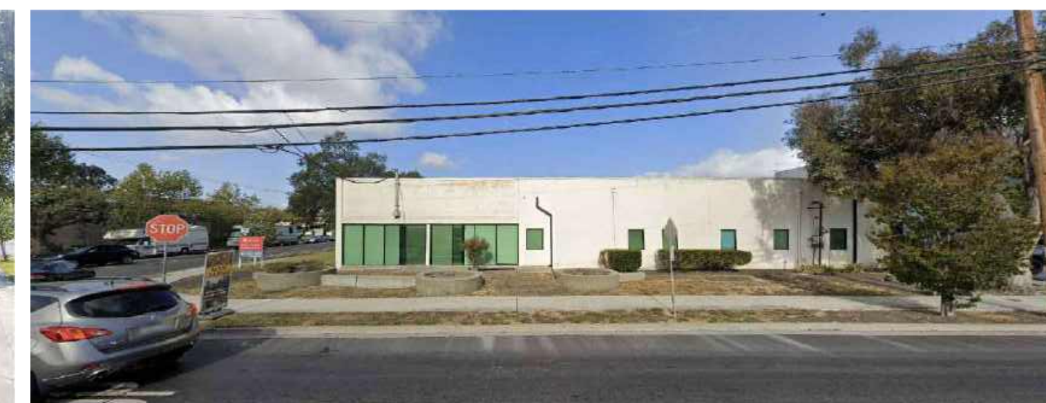
4. VIEW FROM HAVEN AVENUE (EAST)
