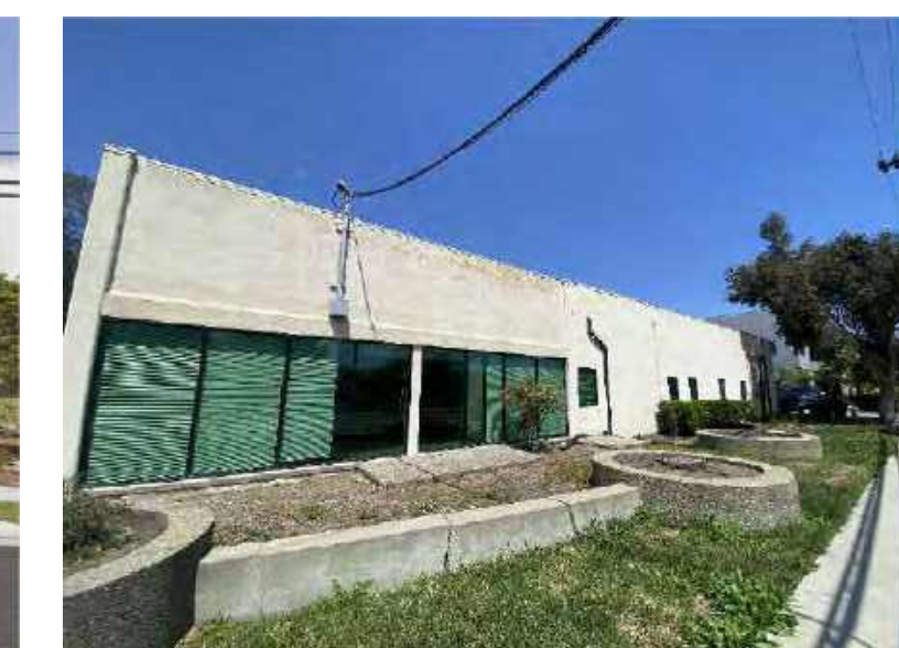
6. VIEW FROM HAVEN AVENUE (EAST), SE CORNER OF SITE
