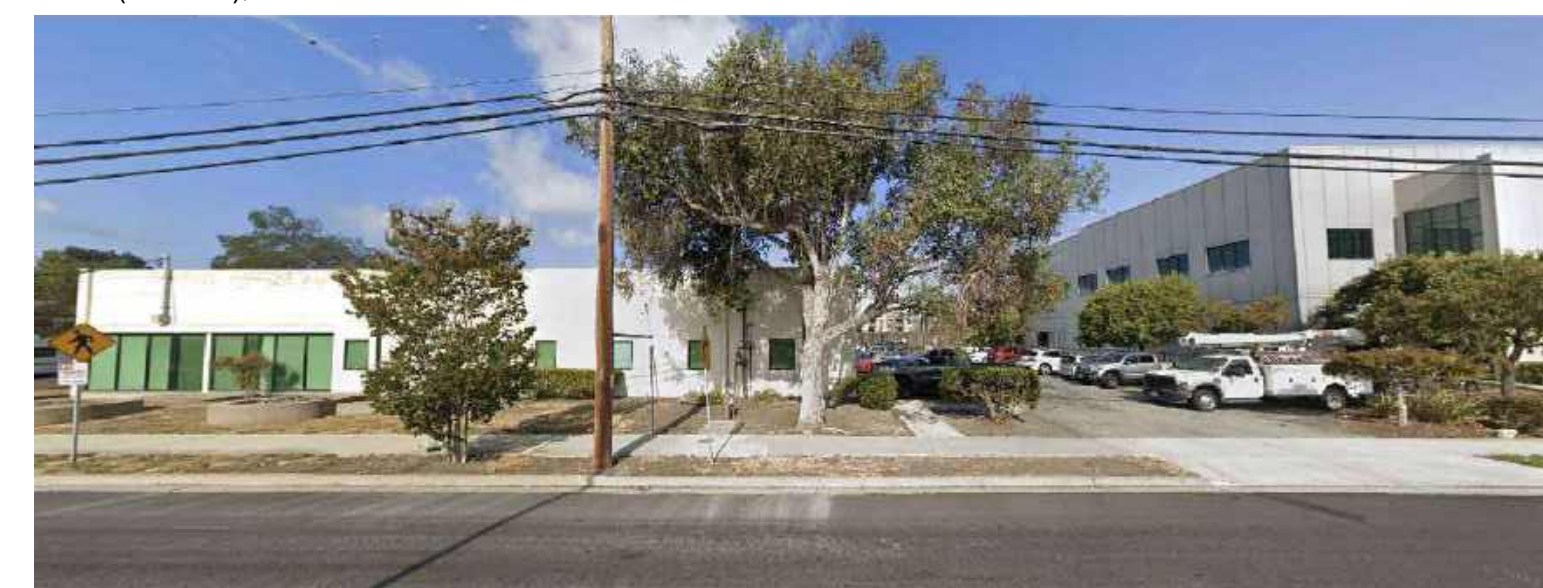
5. VIEW FROM HAVEN AVENUE (EAST)
