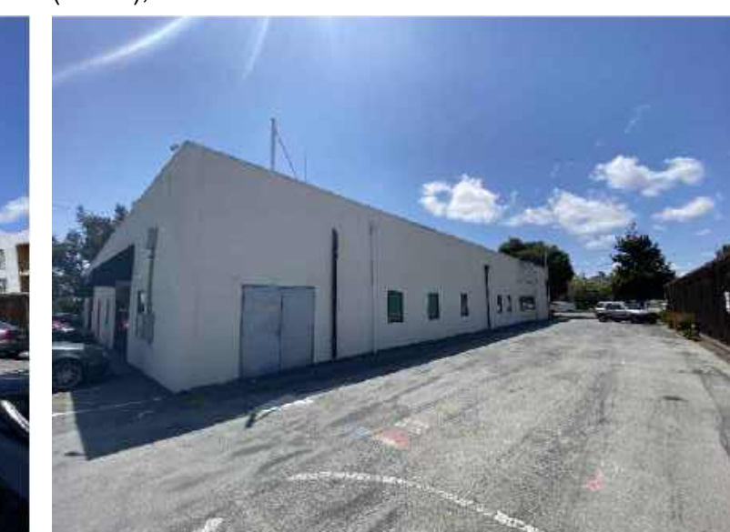
8. VIEW FROM NW PORTION LOOKING SW
