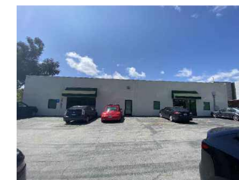
7. VIEW FROM NORTH PROPERTY LINE LOOKING SOUTH INTO SITE
