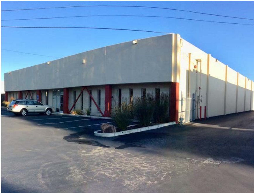
Figure 1: View of South (primary) and East façades, looking northwest. Source: ICF.
