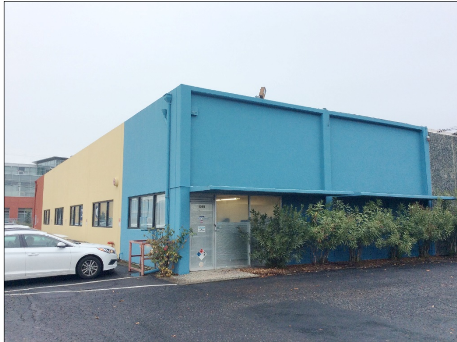
Figure 2. View of south (right) and west (left) facades, looking northeast, 12/11/2019.
