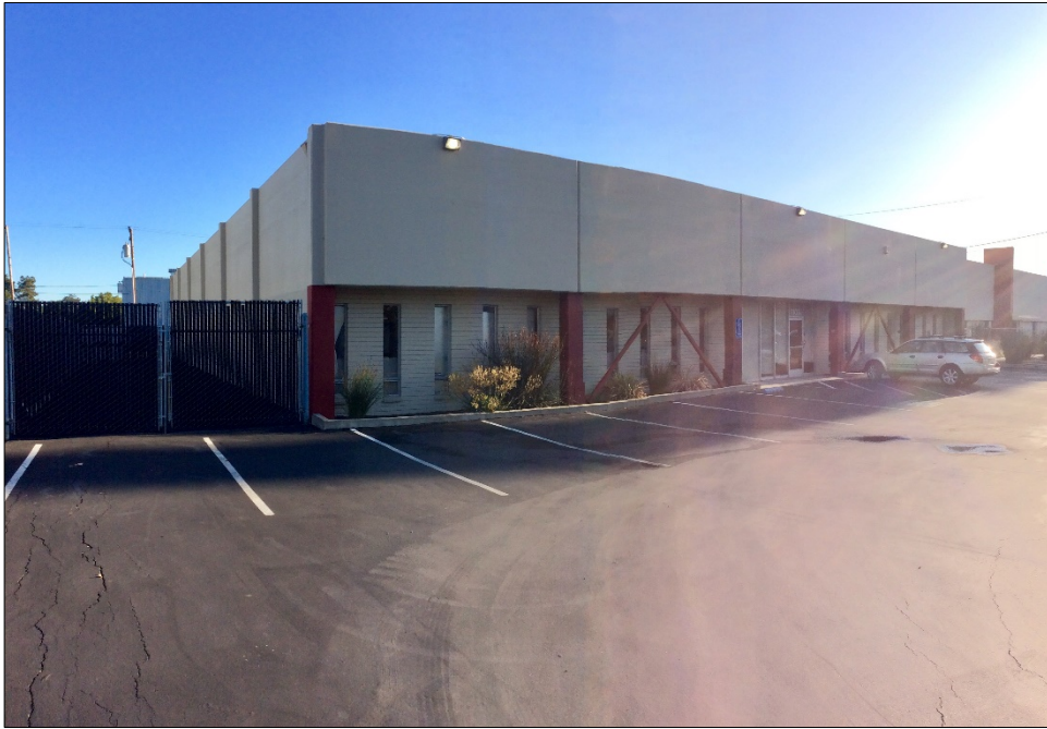
Figure 2. View of south and west facades, looking northeast, 9/20/2018
