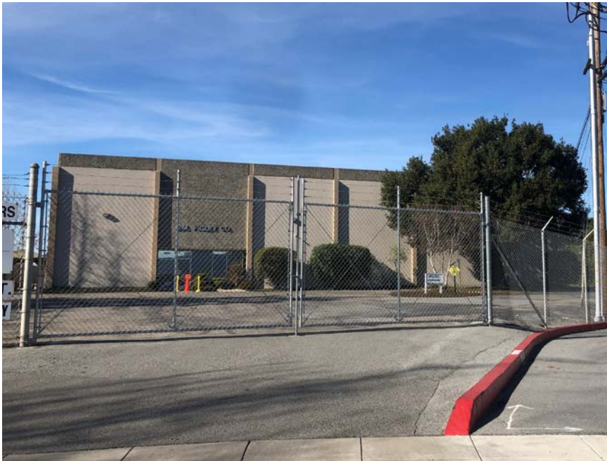
Figure 1: View of west (primary), looking east. Source: ICF.
