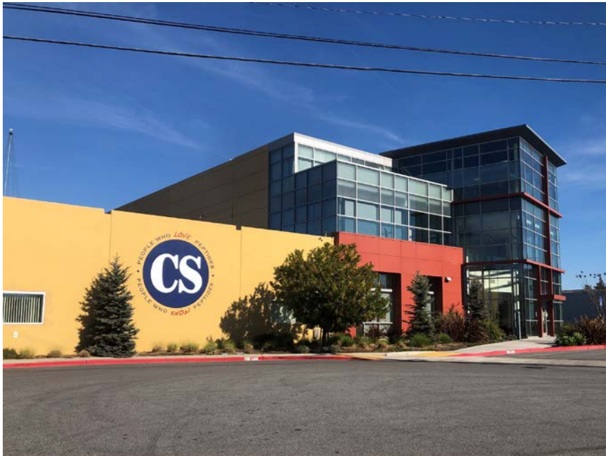
Figure 1: View of south (primary) façade, looking northeast; original building is at left, and 2014 addition is at right. Source: ICF.
