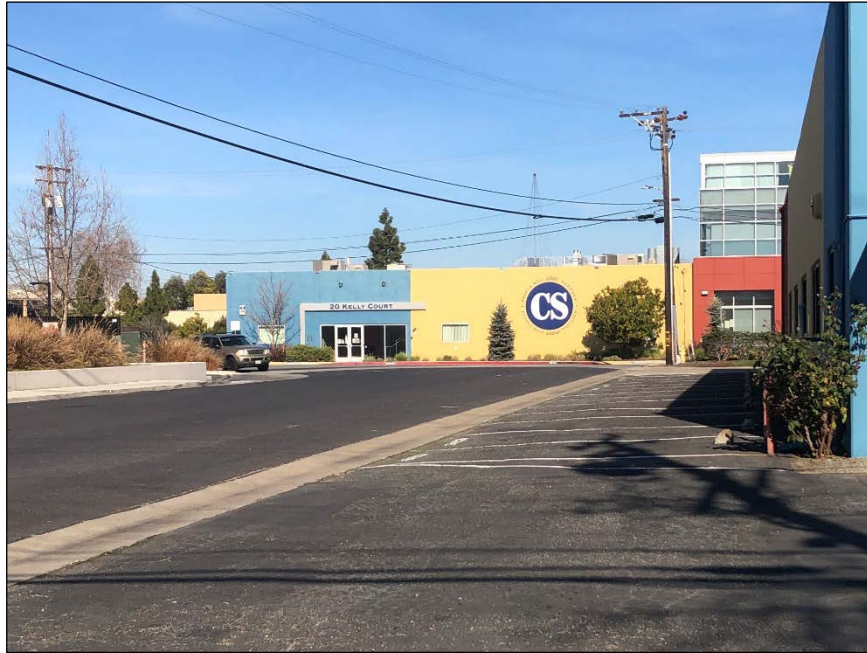
Figure 2. View of the western (original) portion of the south façade, looking north, 1/16/2021.
