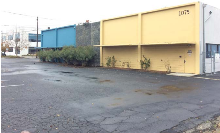
Figure 1: View of South (primary) and East façades, looking northwest. Source: ICF.
