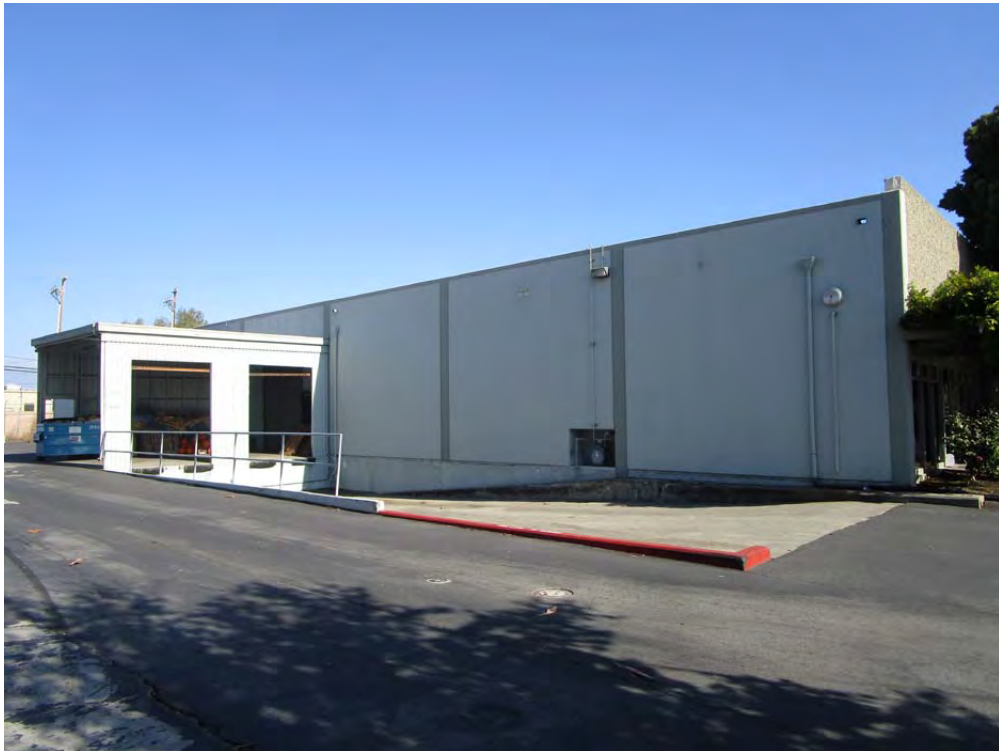
Northwest elevation (left side) of the building at 165 Jefferson Drive
