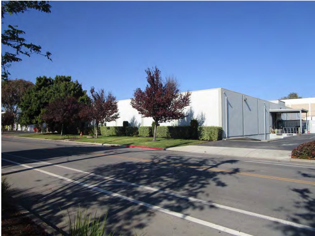
Alternate view of the southwest elevation
