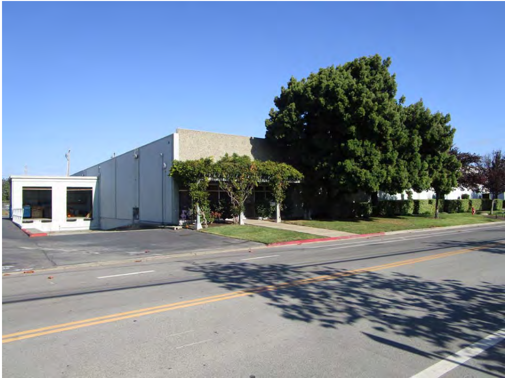
Southwest elevation (front view) of the existing building at 165 Jefferson Drive
