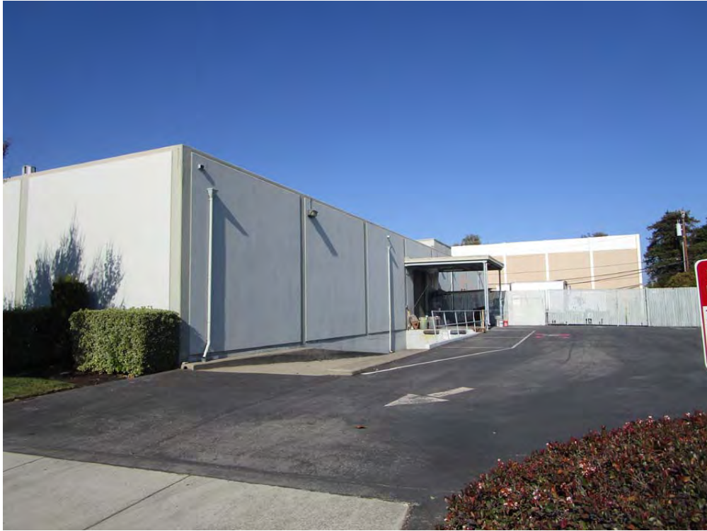
Southeast elevation (right side) of the building at 165 Jefferson Drive
