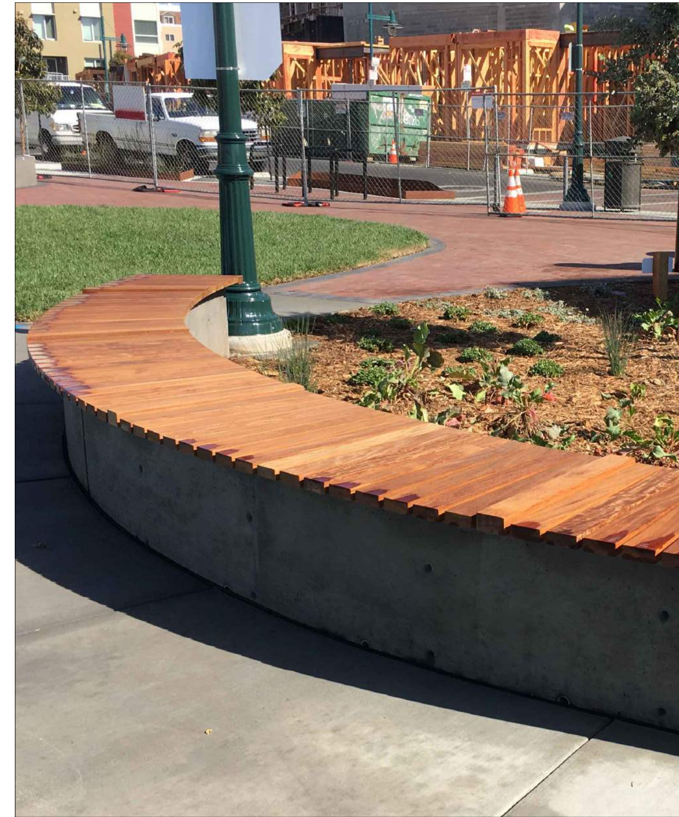
Concrete Seating Steps
