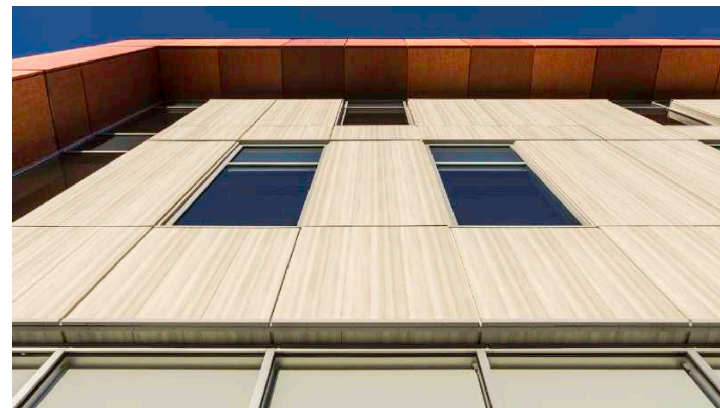
Horizontally oriented, Buff colored, GFRP or Panelized Cement Board
