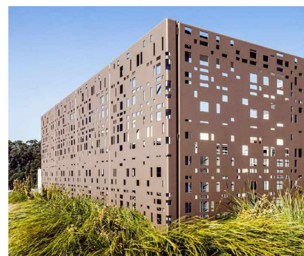
DECORATIVE SCREEN AT BACKFLOW PREVENTERS
