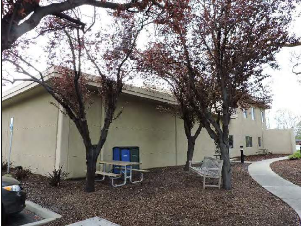
Photograph 6: Northeast façade of 1370 Willow Road (MPK 54), camera facing west, March 27, 2019.
