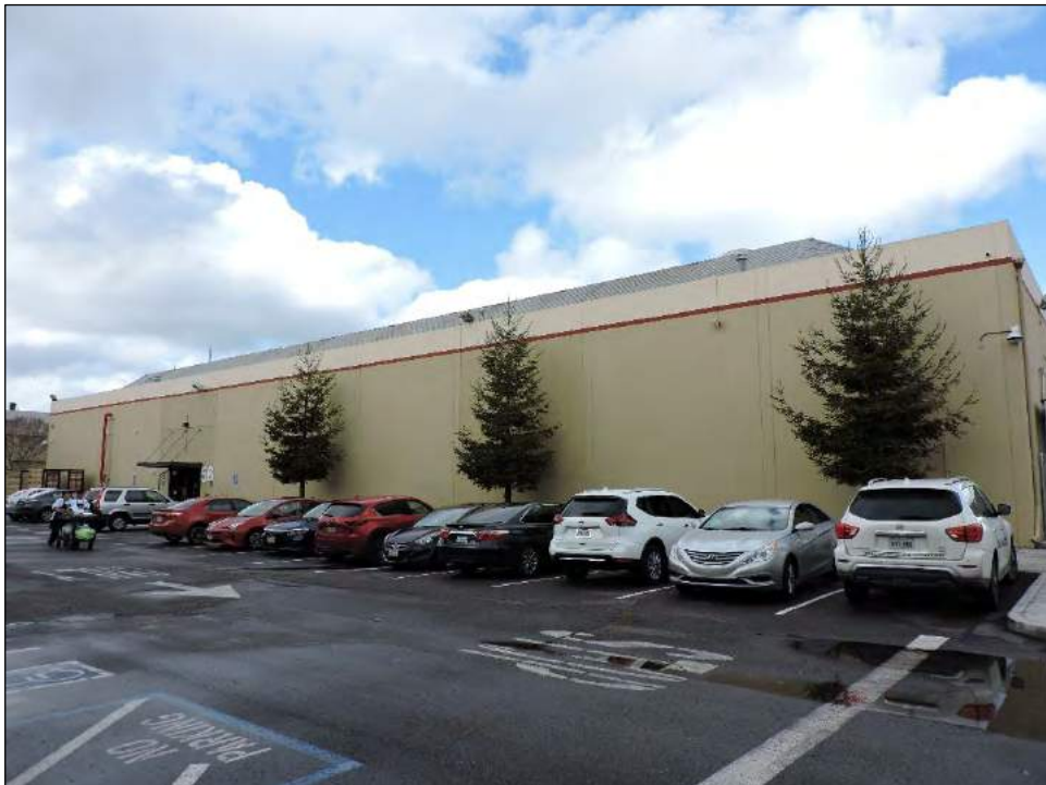
Photograph 19: Southwest façade of 980 Hamilton Avenue (MPK 56), camera facing north, March 27, 2019.
