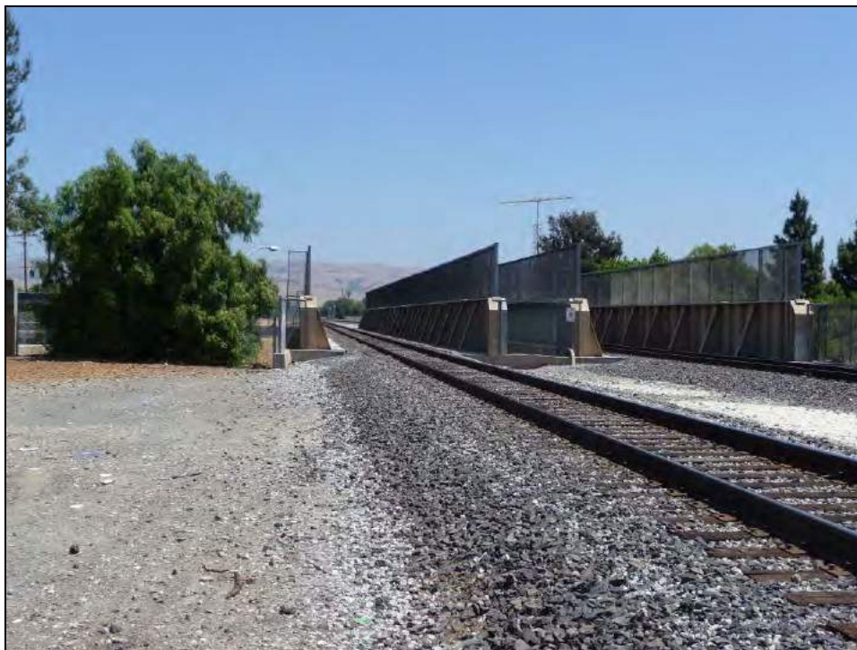
Photograph 6. I-880 Overpass in Fremont, Alameda County, camera facing northeast, 6/16/2008.
