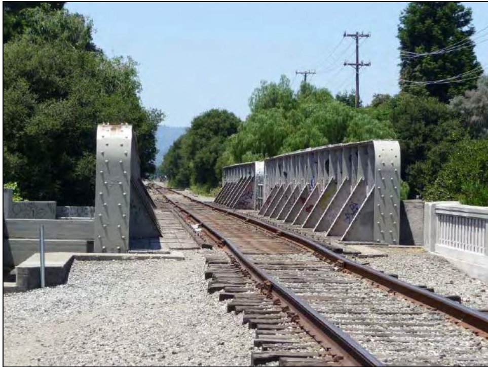
Photograph 3. Showing Henderson overpass, San Mateo County, camera facing east, 6/16/2008.
