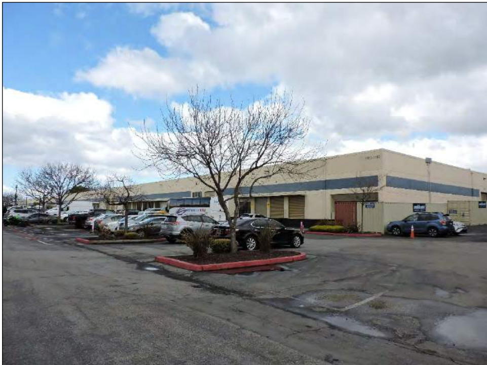
Photograph 23: Typical view of modern buildings within the Willow Village complex, camera facing northeast, March 27, 2019.
