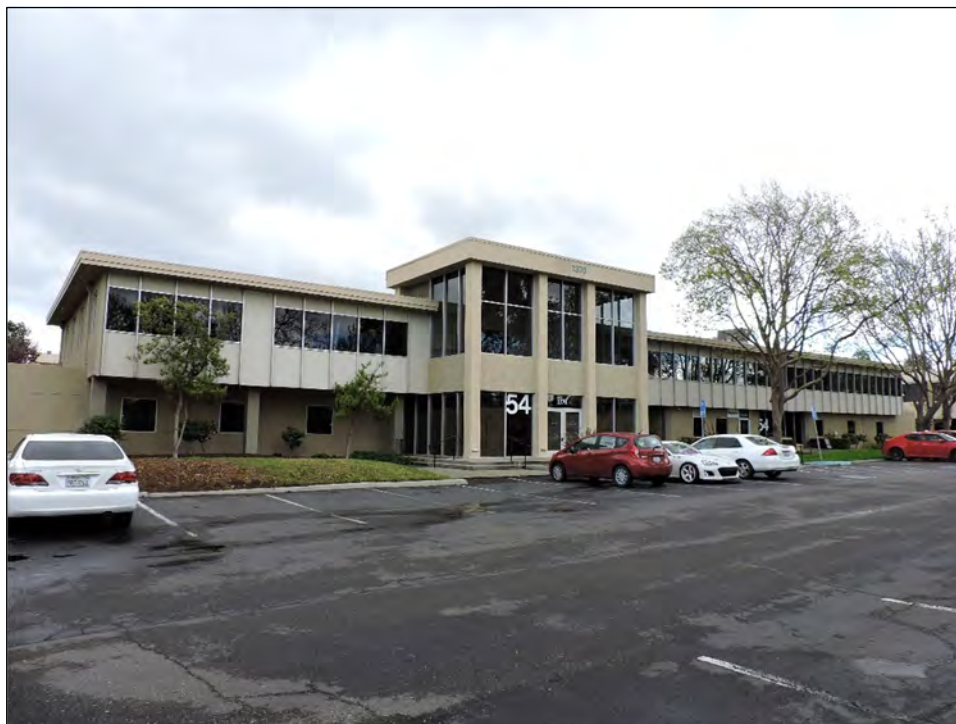
Photograph 5: Primary, northwest façade of 1370 Willow Road (MPK 54), camera facing southeast, March 27, 2019.
