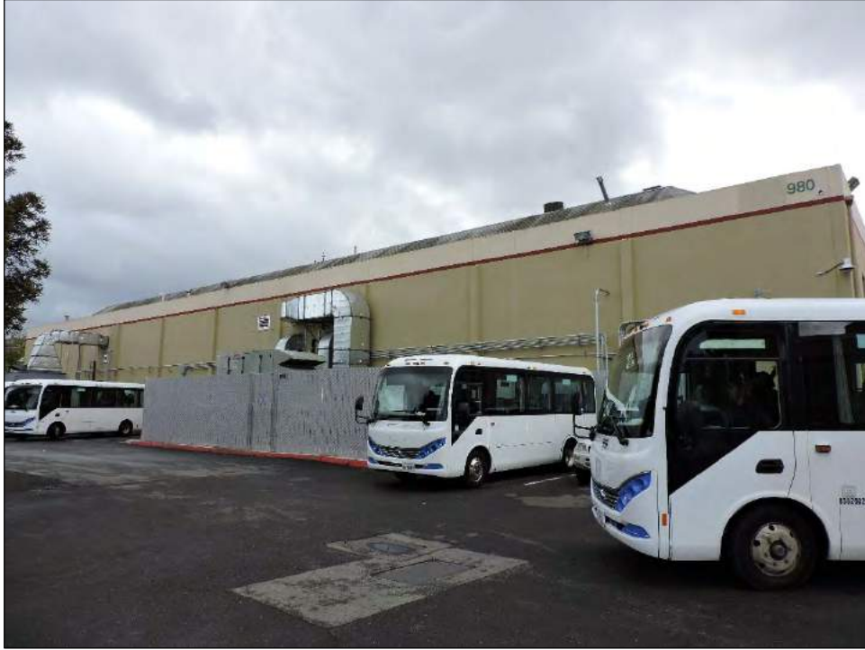
Photograph 22: Northeast façade of 980 Hamilton Avenue (MPK 56), camera facing south, March 27, 2019.
