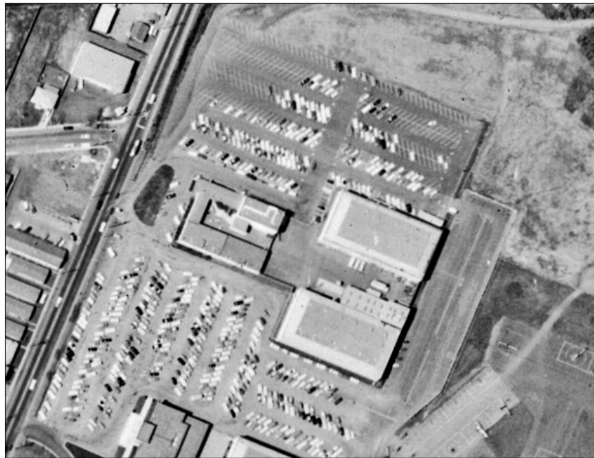
Figure 8. These three buildings at the Hiller Aircraft property were used by Lockheed from 1958 until 1969 for testing and development of the Corona satellites. Note that these buildings were separated from the rest of the facility to the south by fencing. 28
