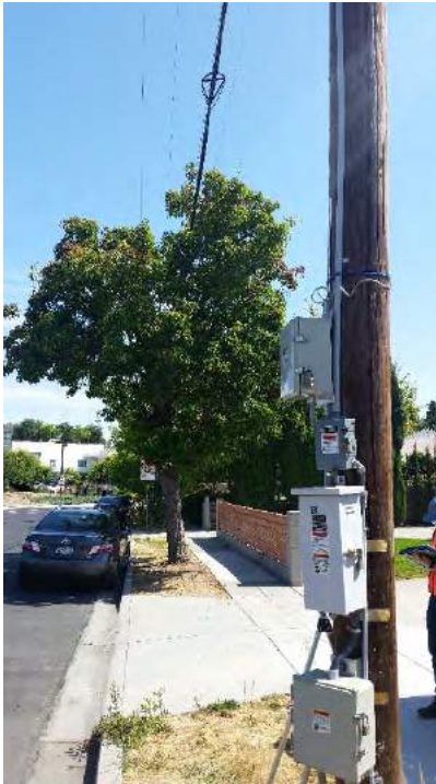
Looking North on Carlton Avenue, ~170 feet South of Hamilton Avenue.
