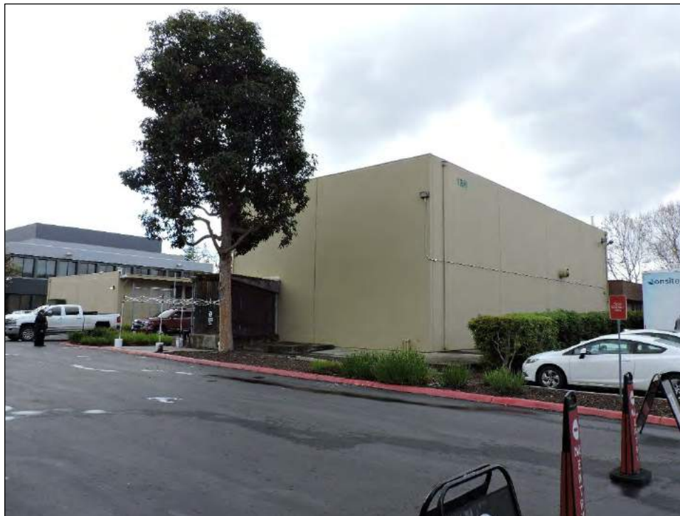
Photograph 4: Unfenestrated warehouse section of 1390 Willow Road (MPK 50), camera facing west, March 27, 2019.
