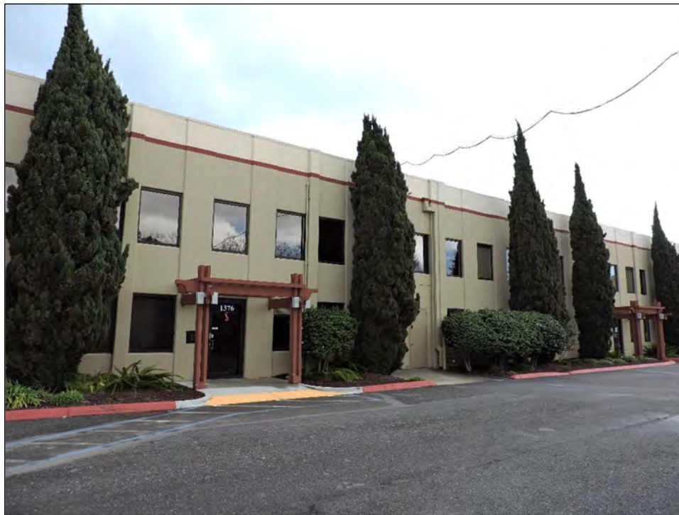
Photograph 10: Northwest façade of 1374 and 1376 Willow Road (MPK 55), camera facing south, March 27, 2019.
