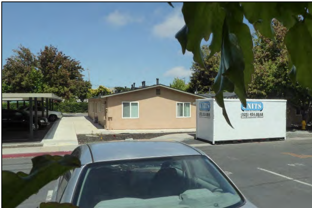
Photograph 2: View of adjacent building 1381 Willow Road (left), with 1385 Willow Road obscured by storage container, at right; camera facing northwest, June 2, 2021.
