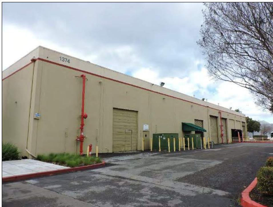
Photograph 13: Southeast façade of 1374 and 1376 Willow Road, camera facing north, March 27, 2019.
