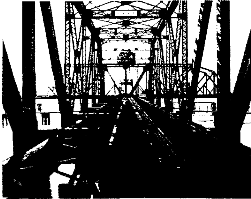
View to southwest through eastern truss approach span 3 toward open draw span, with western approach truss span 4 visible beyond.
