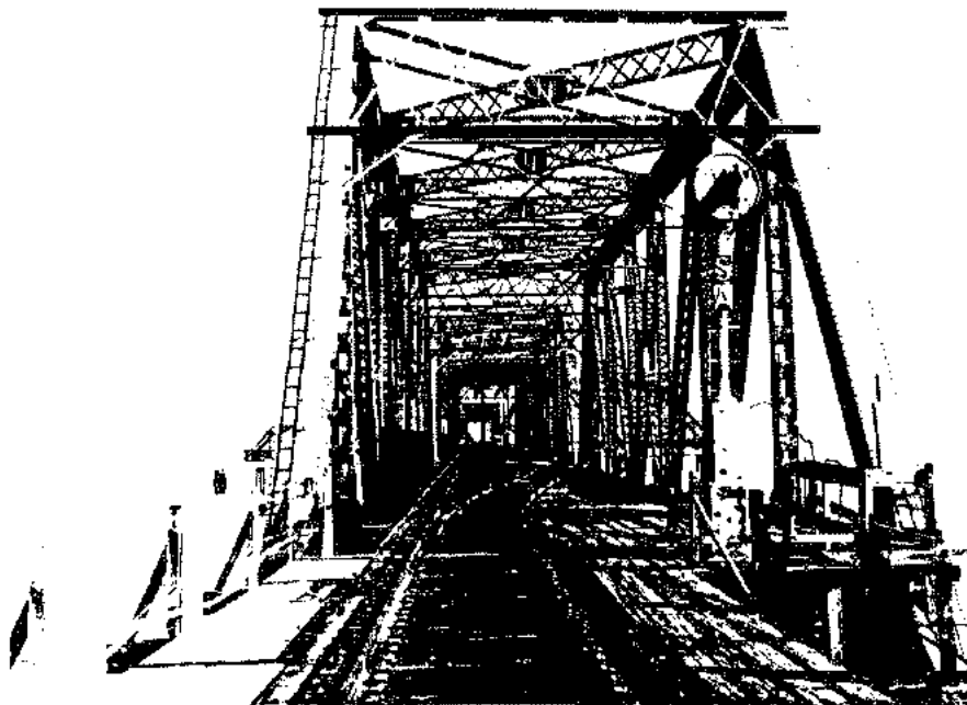
View to northeast of Harriman Common Standard through truss western approach spans (span 6 nearest camera). Note siding on bridge, draw span approach signal at right.
