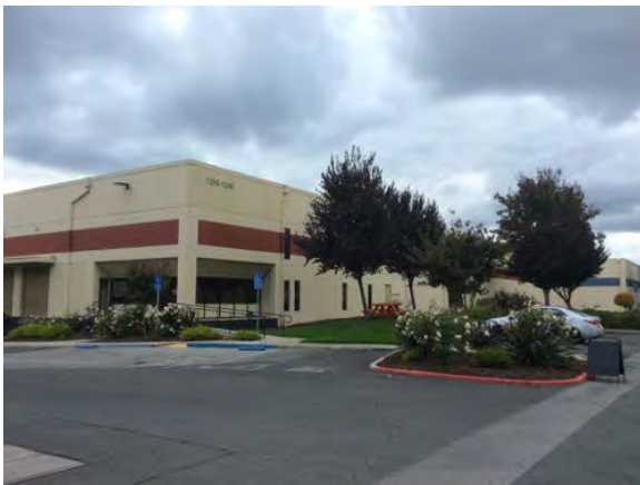
Photo 1. Office buildings, parking lots, and landscape areas on the project site.
