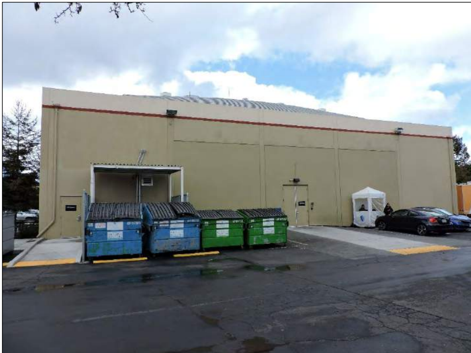
Photograph 21: Southeast façade of 980 Hamilton Avenue, camera facing northwest, March 27, 2019.
