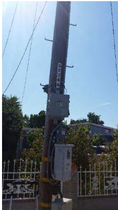
On Carlton Avenue, looking East towards 1396 Carlton Avenue.
