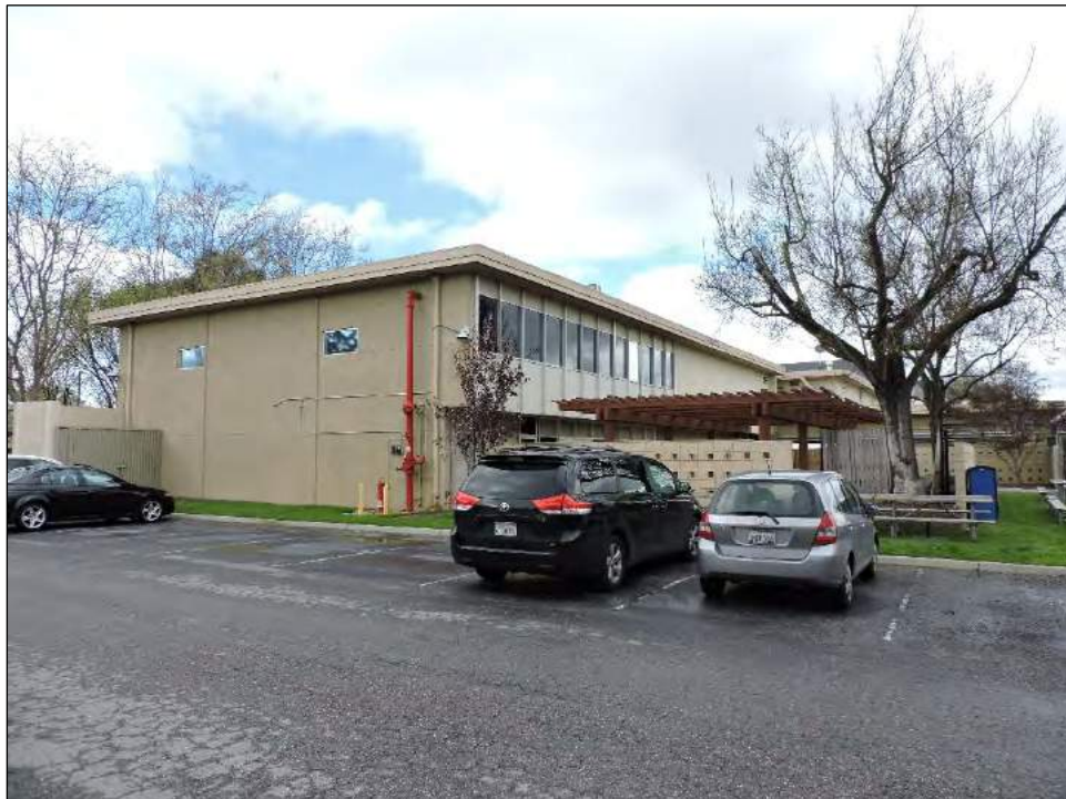
Photograph 7: Southwest façade of 1370 Willow Road, camera facing northwest, March 27, 2019.
