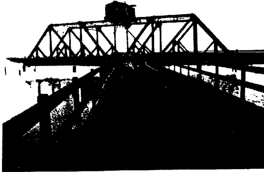
View to southwest of Newark Slough Bridge, from eastern approach.
