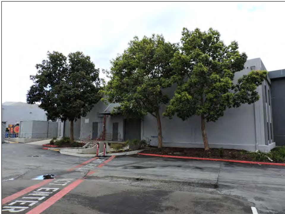
Photograph 15: Southeast façade of 940 Hamilton Court, camera facing southwest, March 27, 2019.
