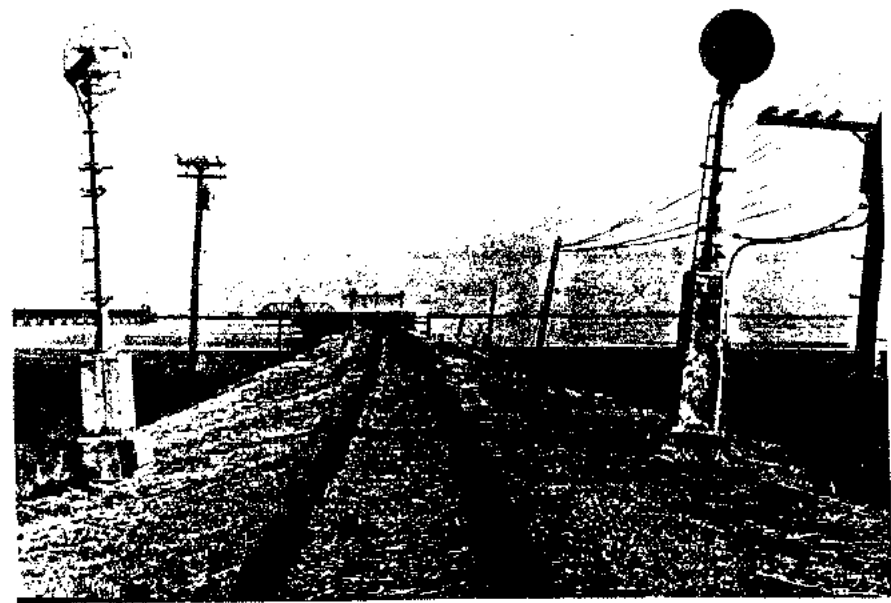
Bridge approach signals, view to northeast toward Dumbarton Bridge. Open draw span visible in distance.
