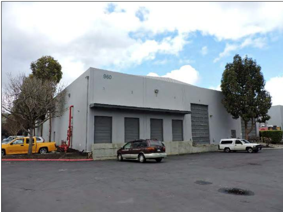
Photograph 17: Overhead freight doors on the southeast façade of 960 Hamilton Court, camera facing northwest, March 27, 2019.
