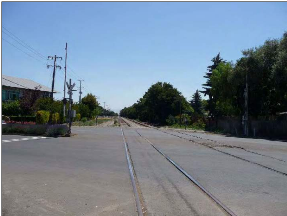
Photograph 2. At Marsh Road in Redwood City, San Mateo County, camera facing east, 6/16/2008.
