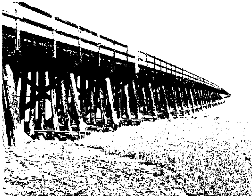
View to north of western timber trestle approach spans, from south side of western abutment.
