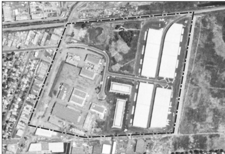
Figure 6. In the early 1980s, Lincoln Properties had begun to make substantial changes to the property by adding new buildings, developing a new road system, and paving parking lots. In this 1982 aerial, the original Hiller plant and its adjacent buildings remained but within a few years they would be demolished and replaced with new office buildings. 23
