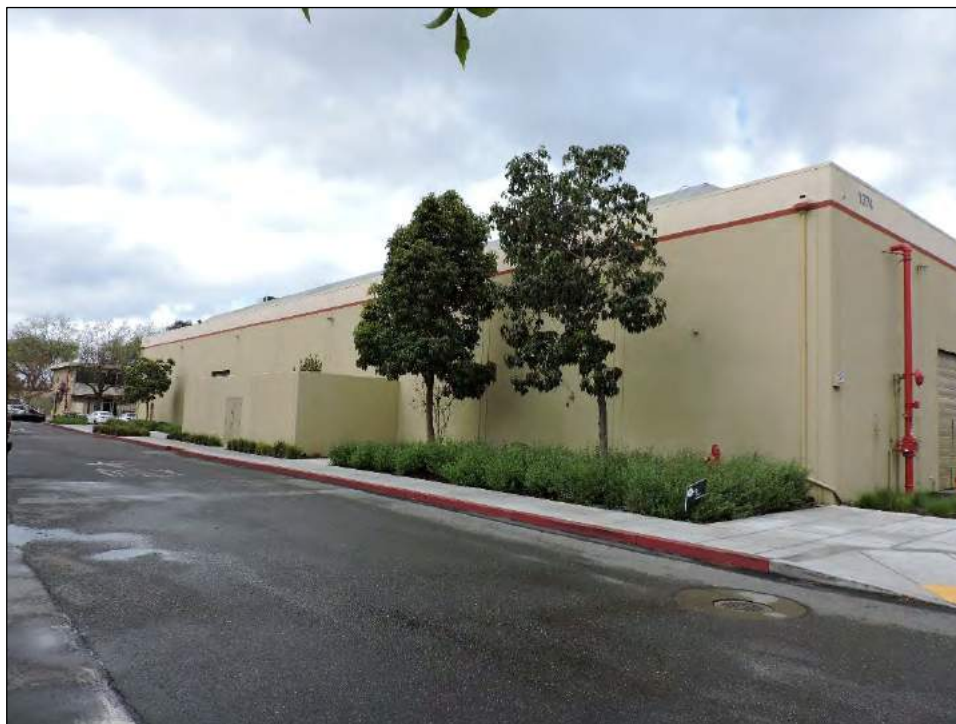
Photograph 11: Unfenestrated southwest façade of 1374 and 1376 Willow Road, camera facing north, March 27, 2019.
