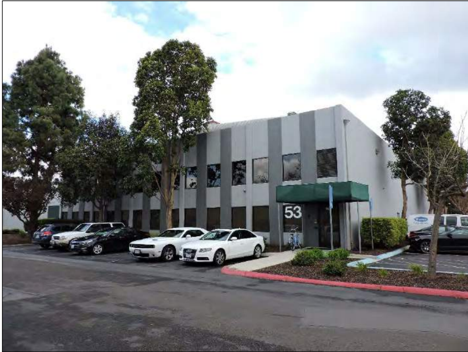
Photograph 16: Northwest façade of 960 Hamilton Court (MPK 53), camera facing east, March 27, 2019.
