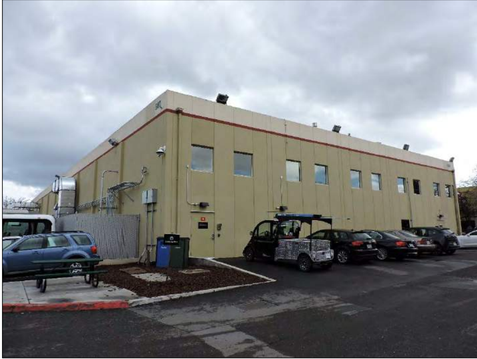
Photograph 20: Northwest façade of 980 Hamilton Avenue (MPK 56), camera facing southeast, March 27, 2019.
