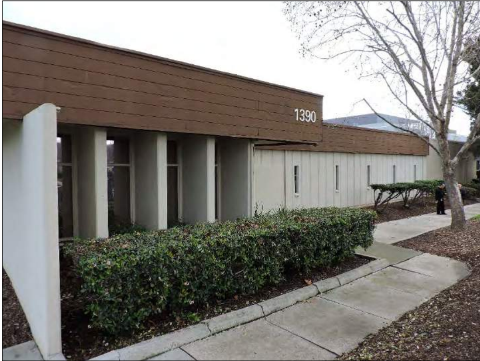
Photograph 2: Northwest façade of 1390 Willow Road (MPK 50), with the entrance vestibule in the foreground, camera facing south, March 27, 2019.
