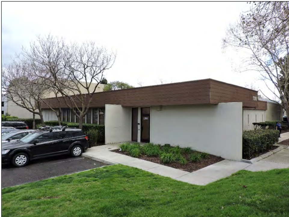
Photograph 3: Northeast façade of 1390 Willow Road, showing the location of a secondary entrance and window ribbon, camera facing south, March 27, 2019.
