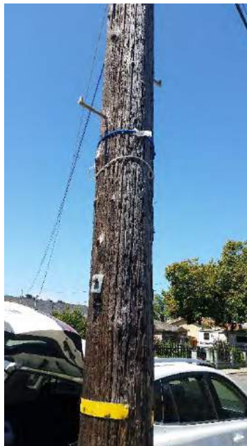
Looking Southwest along Alberni Avenue.
