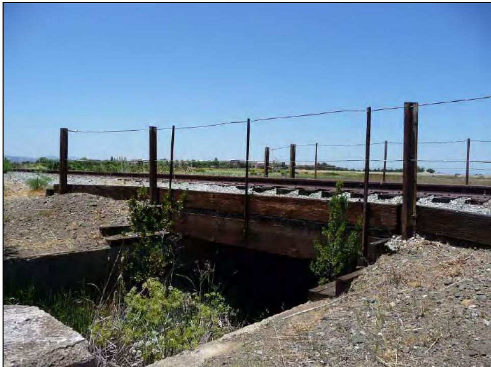
Photograph 8. Showing culvert west of University Avenue, camera facing southwest, 6/16/2008.
