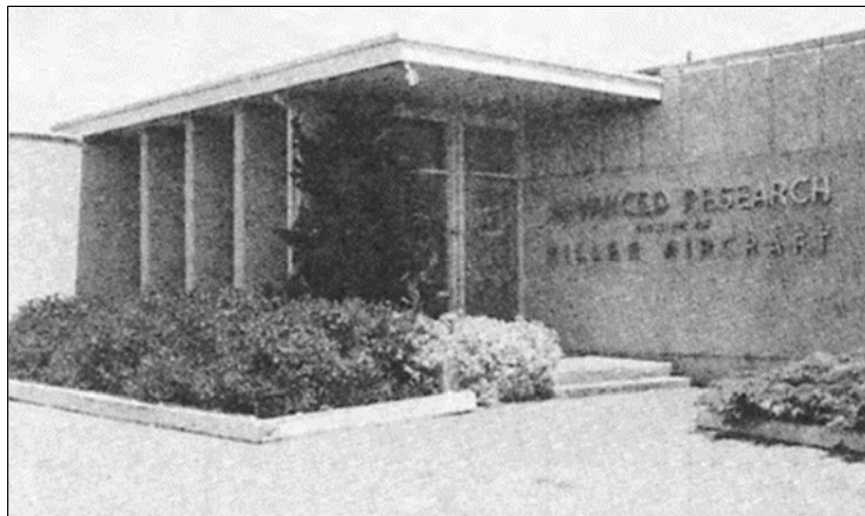
Figure 7. From 1958 to 1969, the Hiller Aircraft Advanced Research Division building was used by Lockheed Corporation to develop the Corona surveillance satellites. As a highly guarded secret, the program did not change the appearance of the building, which retained the Hiller Aircraft signage, as seen in this photograph. The signage has since been removed. 26
