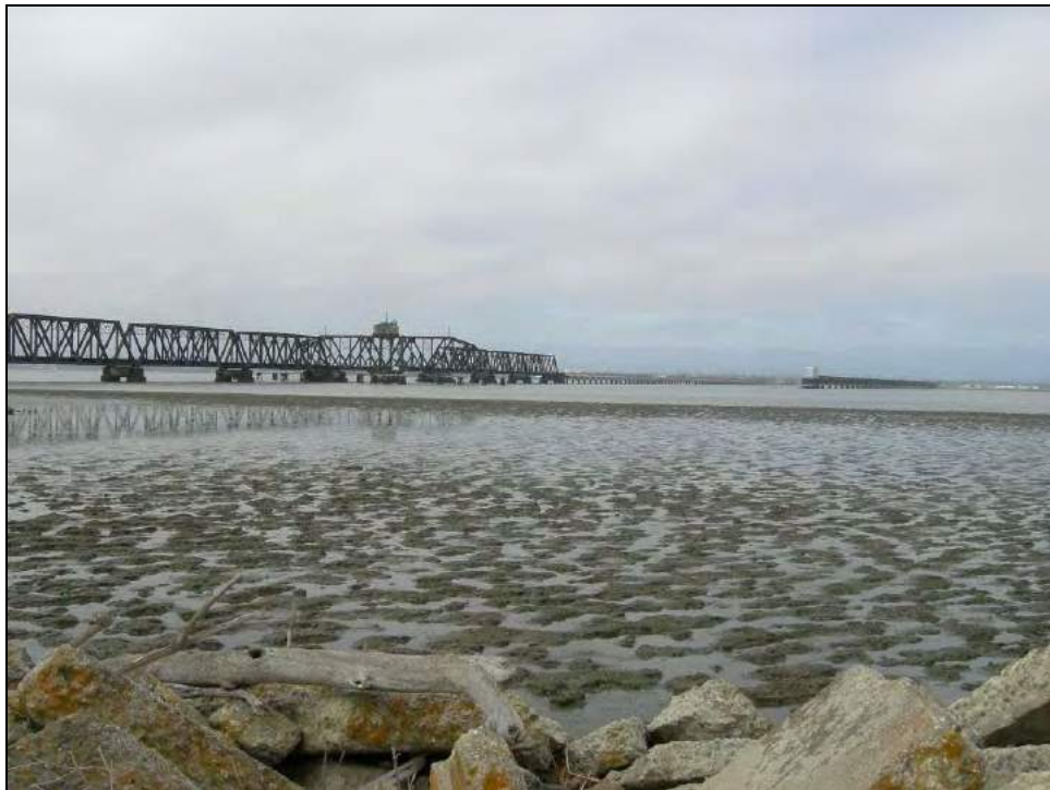
Photograph 4. Dumbarton Bridge over San Francisco Bay, camera facing southwest, 6/16/2008.
