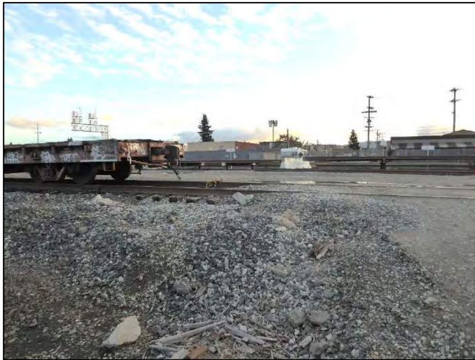
Photograph 1: View of Dumbarton Cutoff where it splits from the mainline; camera facing south, January 25, 2017.
